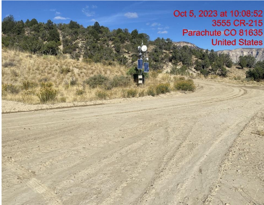
Insufficient Vehicle Tracking BMPs at Location Entrance/Exit – Photo #06818
