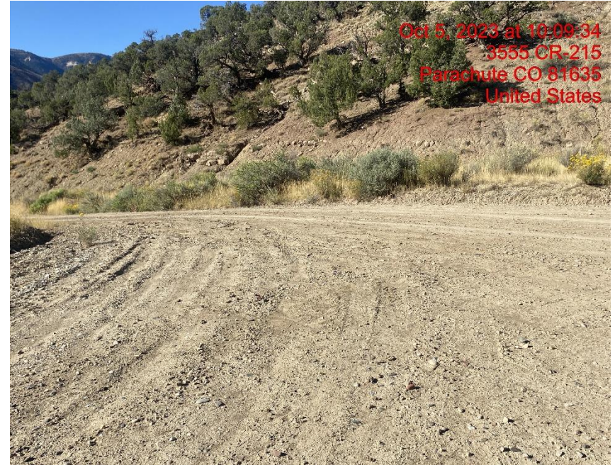
Insufficient Vehicle Tracking BMPs at Location Entrance/Exit – Photo #06819
