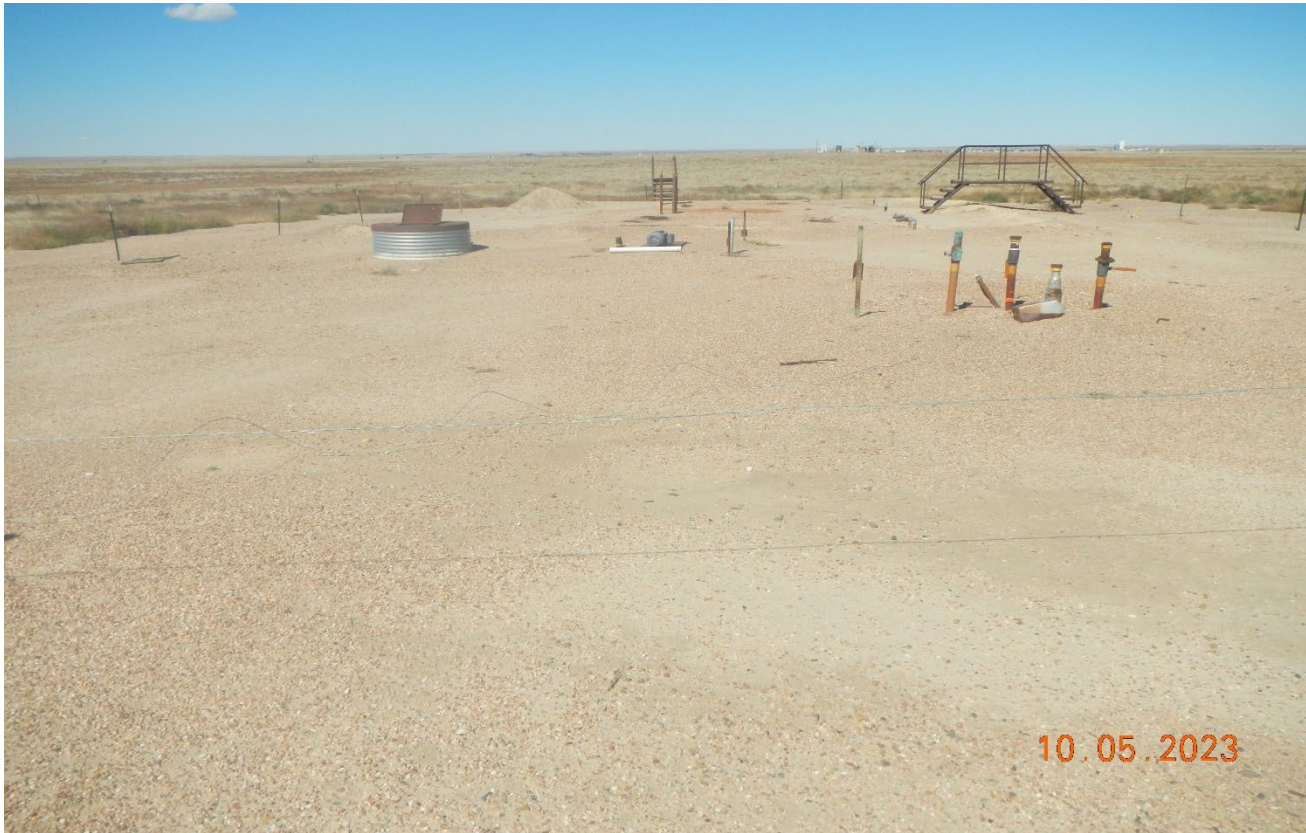
Photo 3. Facing toward the tank battery site. The tanks have been removed however, unused pipe risers and various equipment still remains.
