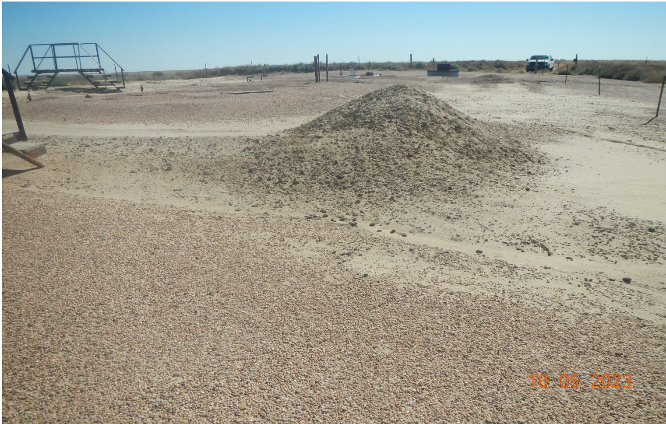
Photo 6. Facing toward the southeast. There is Stormwater erosion occurring off this area of the location. It appears impacted soils have been pled up and are not properly contained.
