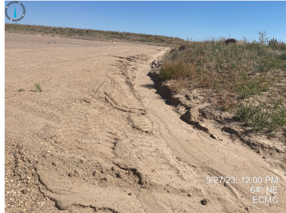
Photo 24. Taken from the southern portion of the production area. Erosion degradation observed from the unstabilized production areas.
