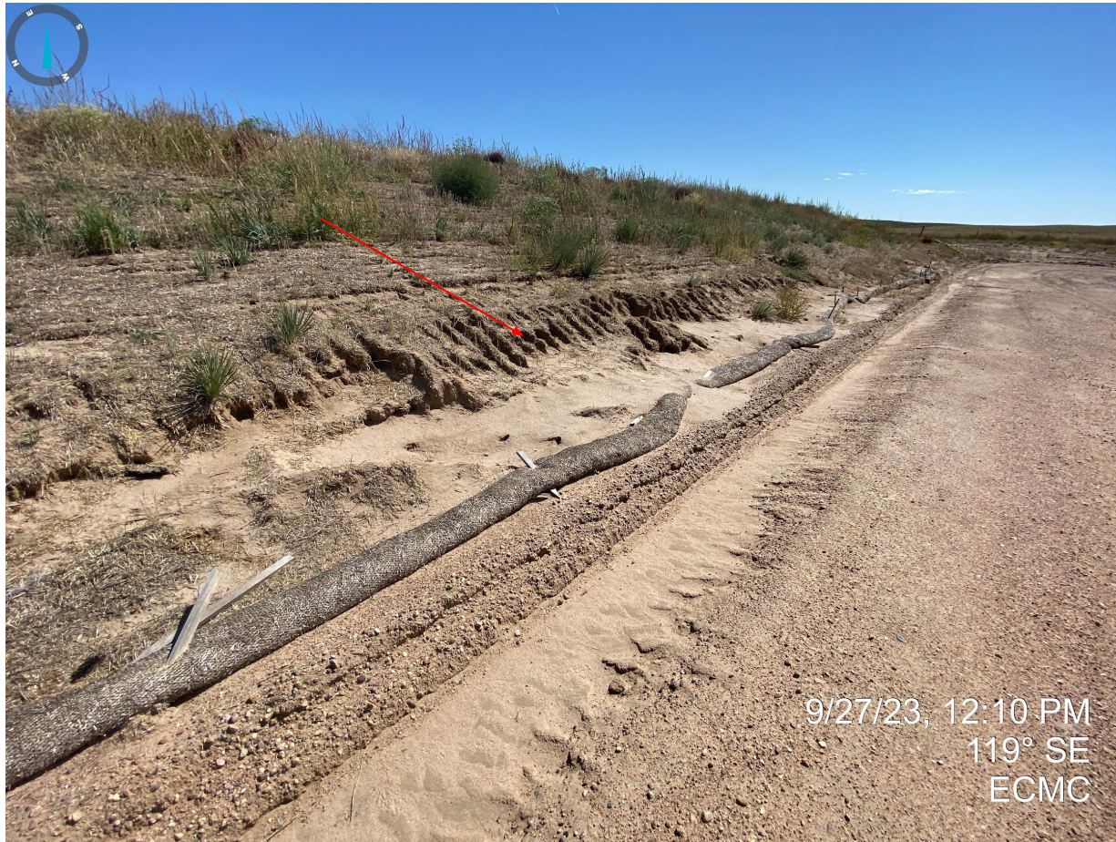
Photo 33. Taken from the western side of the topsoil stockpile. Erosion degradation and sediment transport was observed for the improperly stabilized stockpile. Stormwater control measures( straw wattles) are inadequate as they are beginning to fill with sediment, not installed correctly, and starting to degrade.
