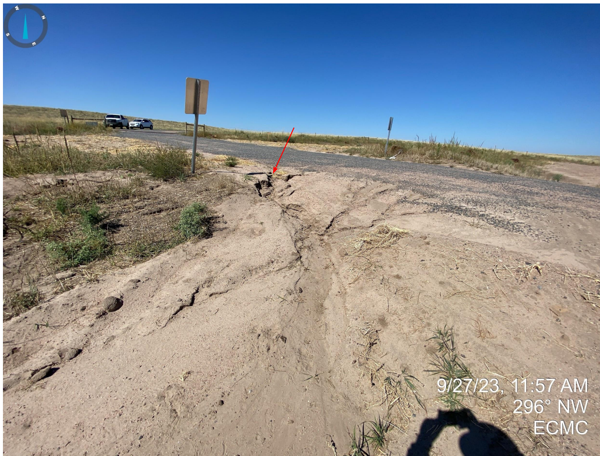
Photo 19. Taken from the sediment trap on the western side of the production pad. Rill and gully erosion degradation evident. Stormwater control measures do not appear to be adequate for this location as unstabilized soils were observed.
