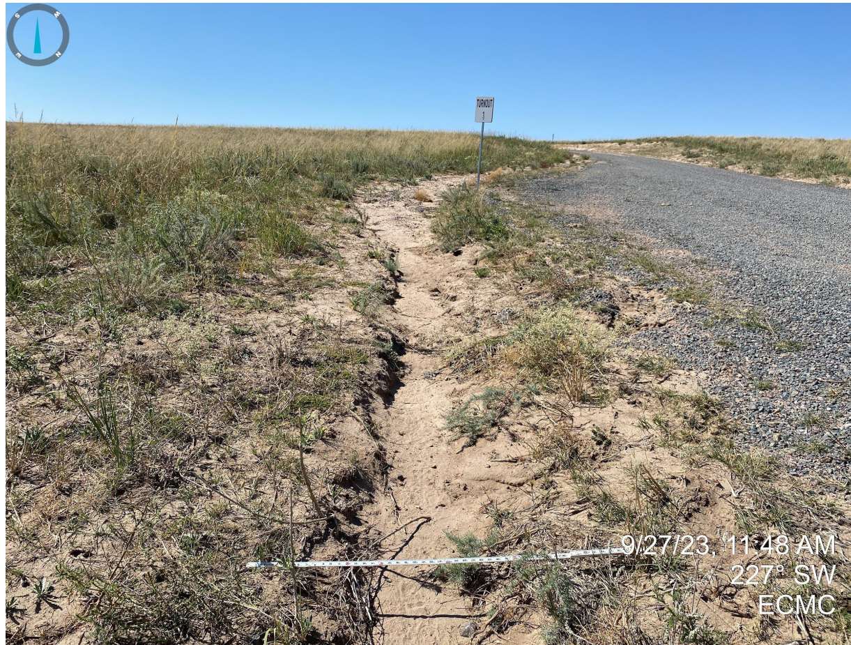
Photo 10. Southside of access road, approximately ¼ mi west of the location. Gully erosion degradation pictured; no apparent stormwater control measures/BMPs observed.
