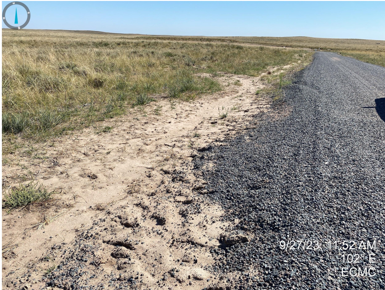
Photo 14. Taken approximately 500' west of the location. Offsite sediment transport; no apparent stormwater control measures observed.
