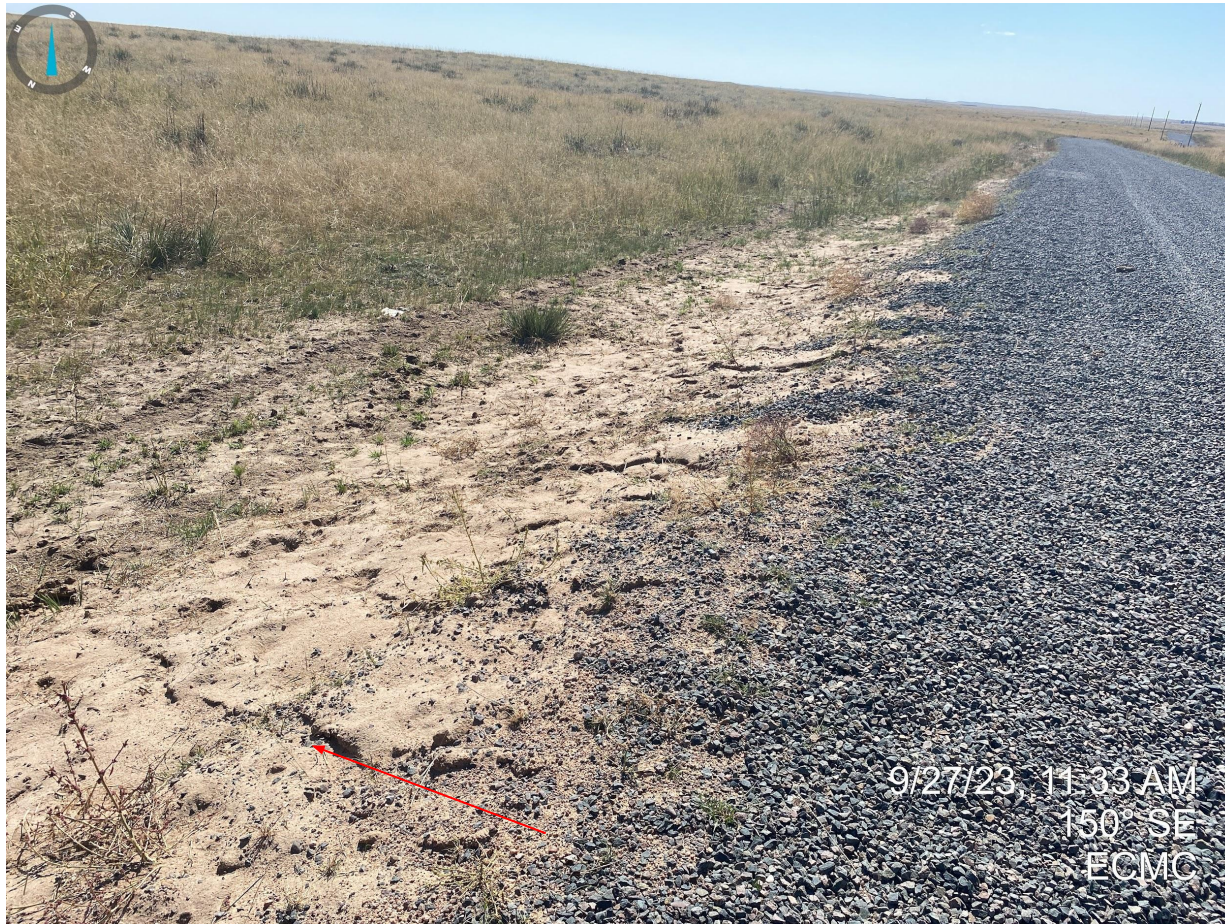
Photo 2. Taken approximately 1 mile north from the entrance. Rilling degradation was observed on the shoulders of the access road, indicating that the disturbance areas are not properly stabilized from wind and water erosion.
