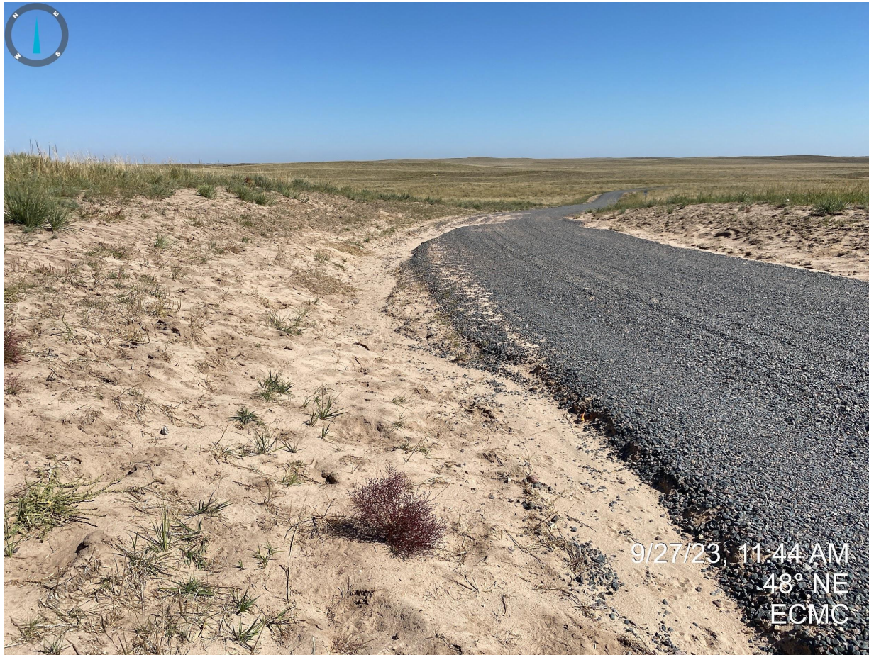
Photo 6. Taken approximately ¼ mile west of the location. Photo illustrates that cut banks are not properly stabilized with evidence of bare/exposed soils and and erosion degradation occurring.
