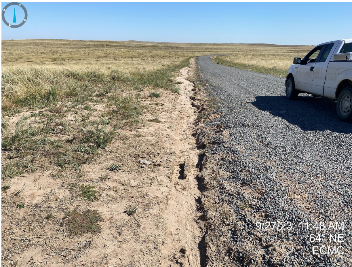
Photo 9. See comments in Photo 6. No apparent stormwater control measures observed along the access road/ditch.
