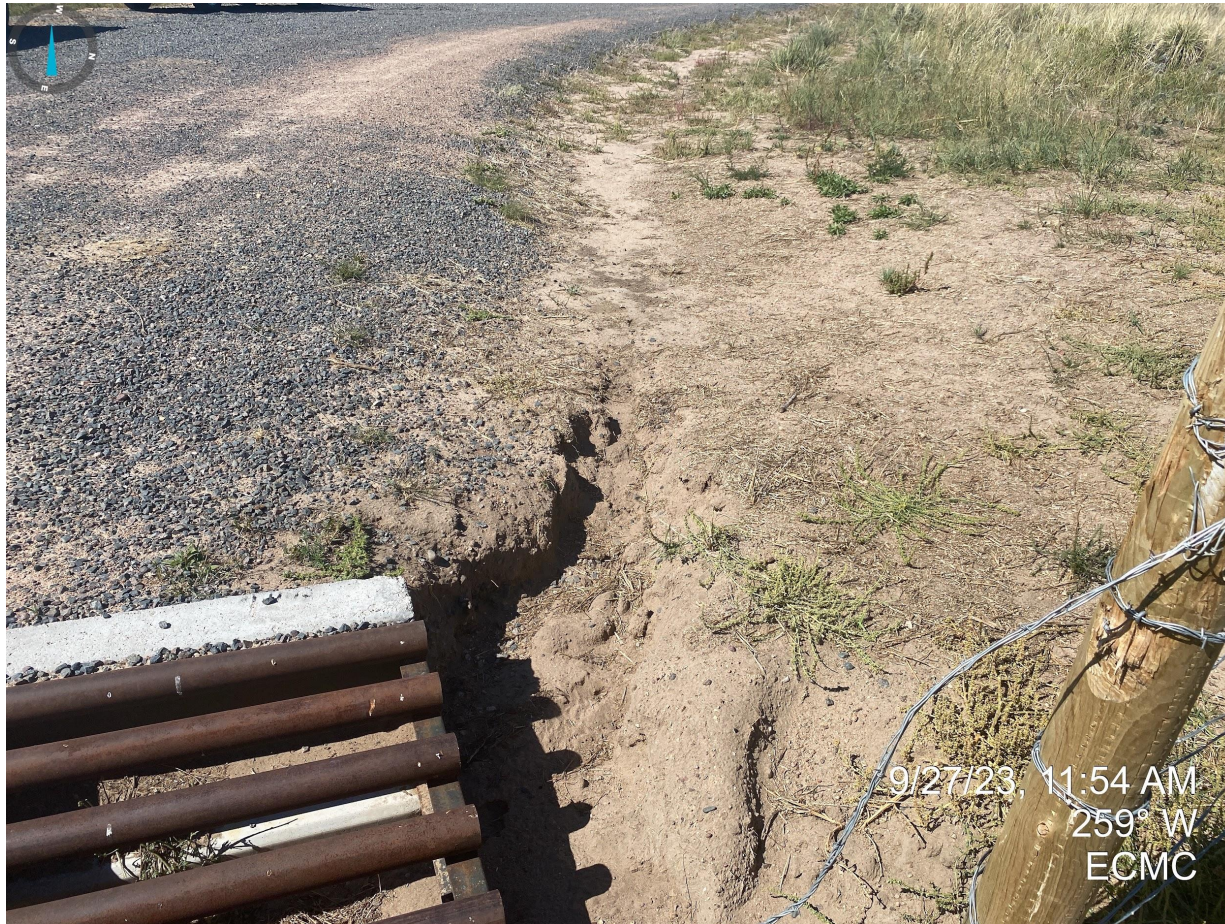
Photo 15. Taken at the location's entrance. Erosion degradation occurring at the cattle guard.
