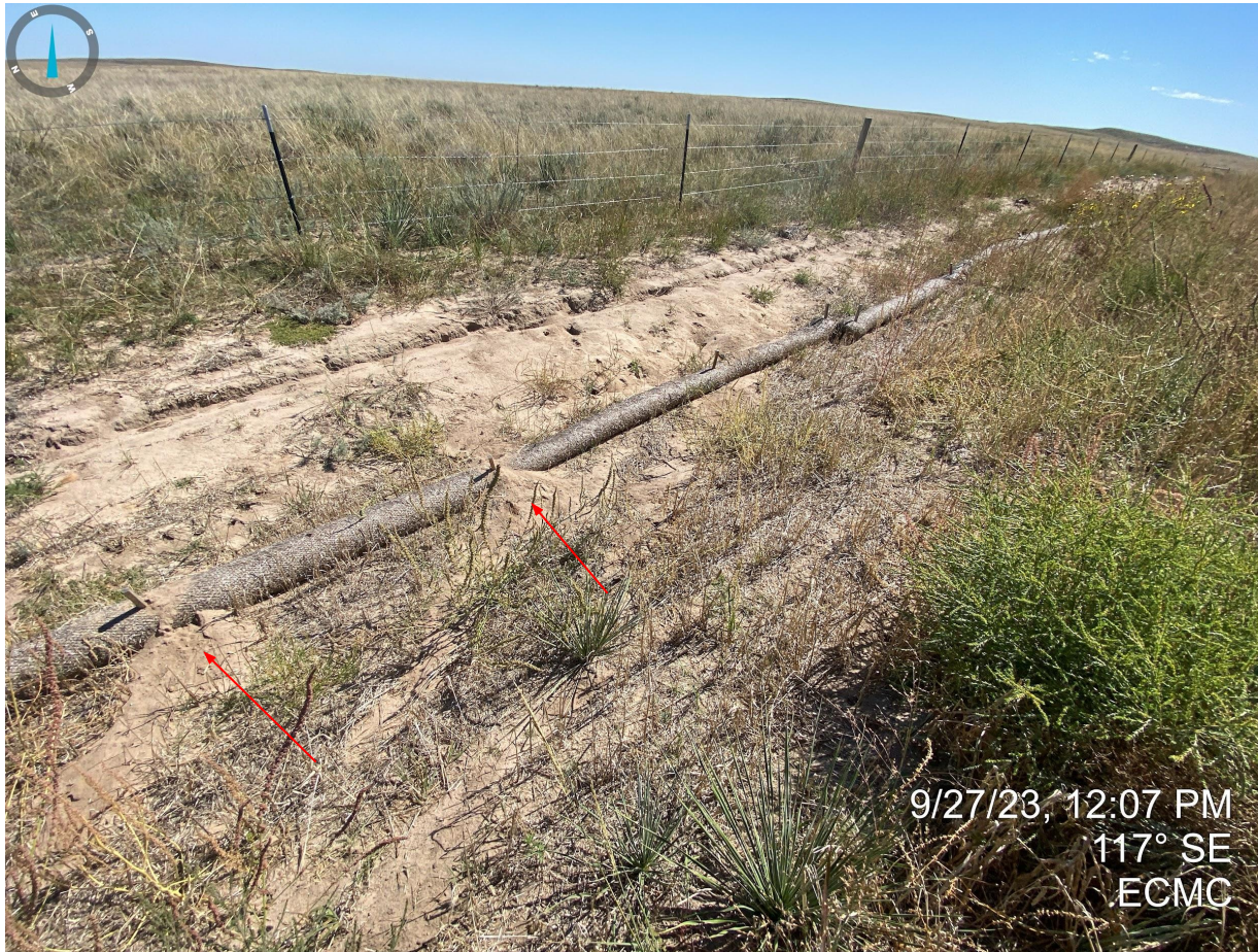
Photo 30. Taken from the eastern side of the topsoil stockpile. Stormwater control measures are not properly installed and are beginning to degrade; evidence of sedimentation around the wattles was also observed.
