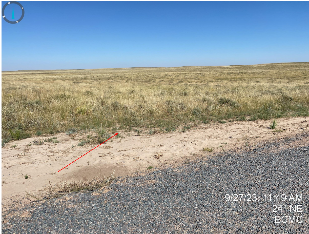
Photo 12. North side of the access road, approximately 1000' west of the location. Photo illustrates that sediment transport is beginning to migrate onto adjacent lands with no apparent stormwater control measures observed.
