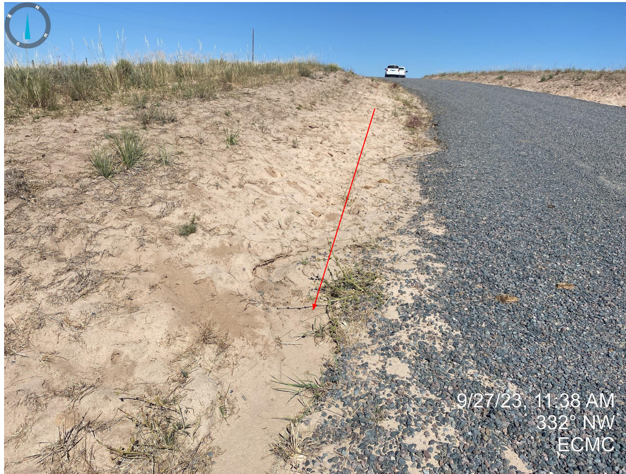
Photo 4. Taken approximately 1 mile north of the entrance. Photo illustrates that cut banks are not properly stabilized with evidence of bare/exposed soils and and erosion degradation occurring.
