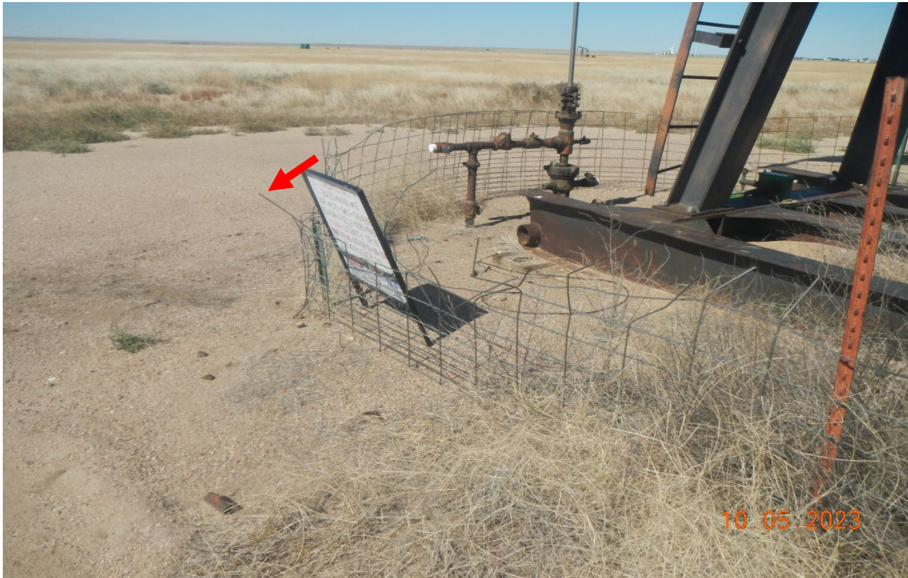
Photo 8. The fence around the pumpjack is not adequate to prevent livestock entry and is only 2ft. Tall near the well sign. There are wires stick out (red arrow) which could injury livestock..
