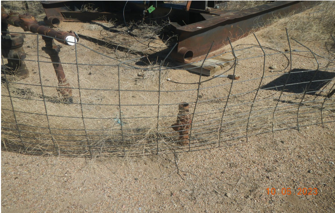
Photo 7. There is an open pipe riser that needs OOSLAT or needs to be removed.
