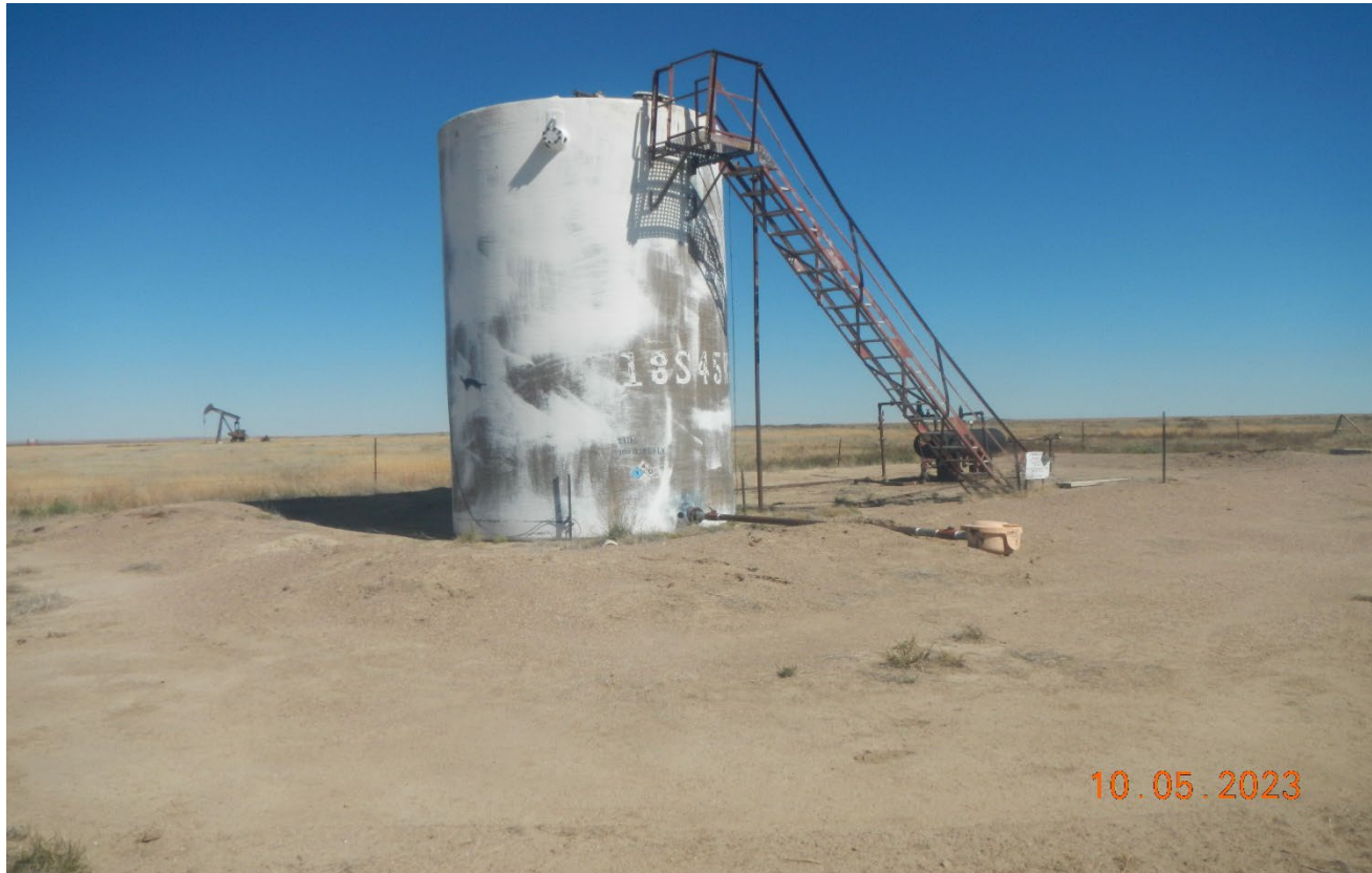
Photo 1. Facing northeast toward the tank battery. Berm is not adequate for containment.
