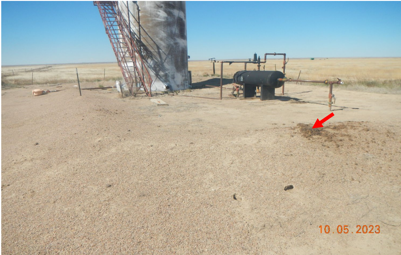
Photo 3. The berm around the tank is insufficiently sized to contain a spill./ There is oily contaminated soils on the berm (red arrow) that needs to be cleaned up and removed.
