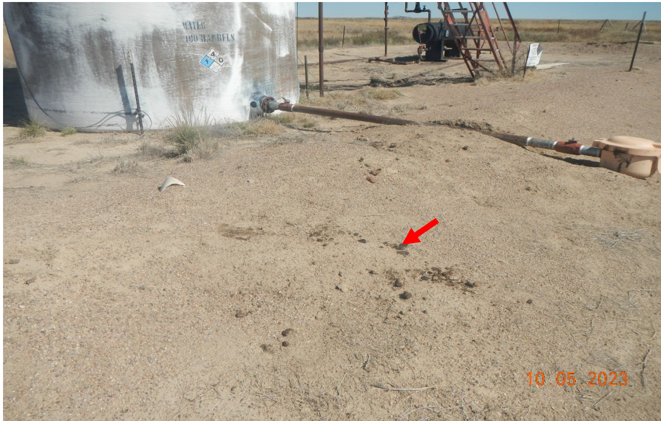
Photo 2. The pipe has been reinstalled at the tank however oily stained soil still remain.
