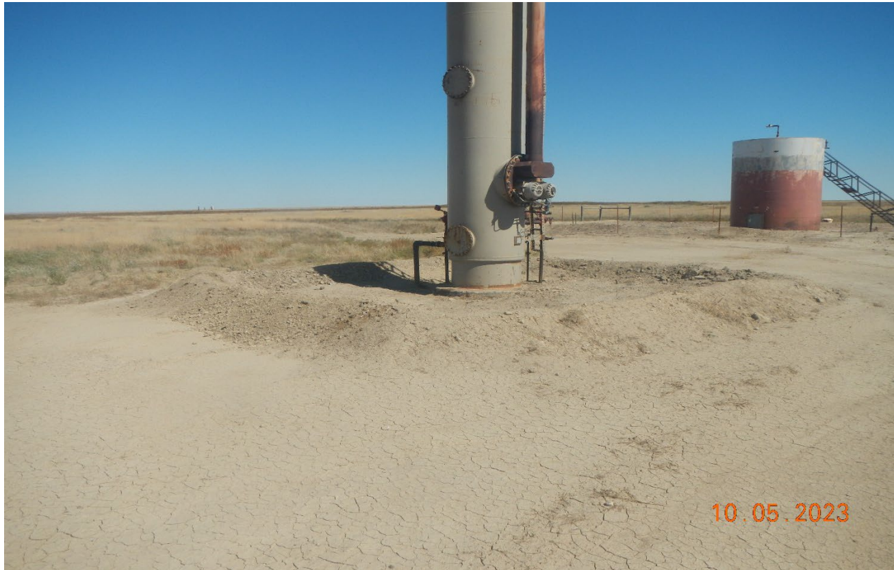
Photo 5. Facing northeast toward the separator. A berm was placed around the separator however the earthen berm is not properly built.
