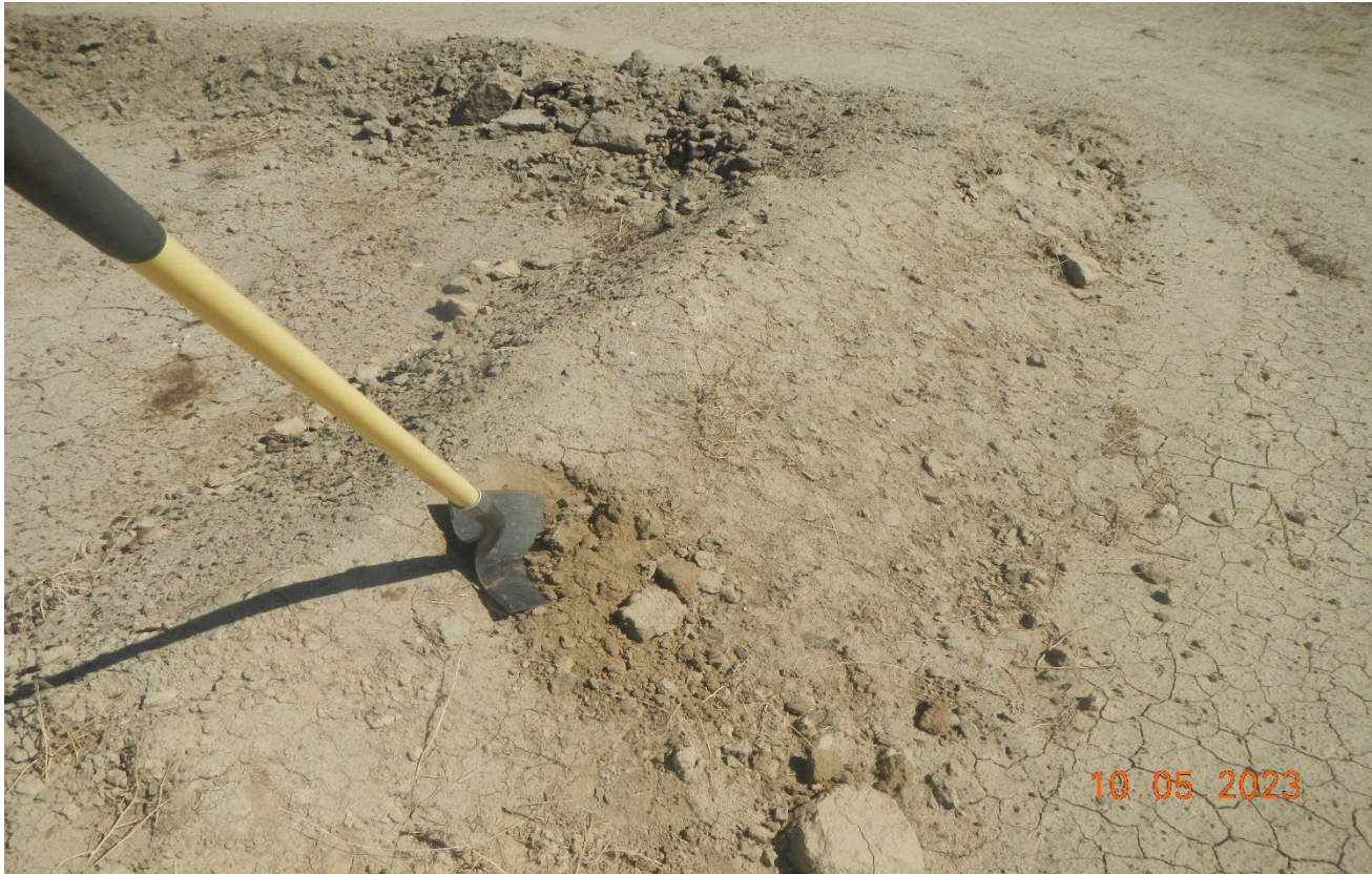
Photo 6. The berm around the separator is not compacted and built sufficiently for containment.
