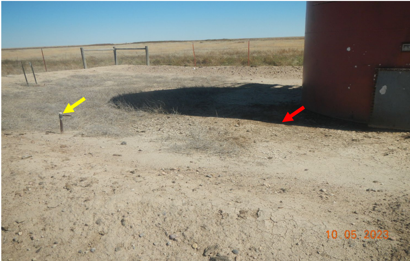
Photo 9. There is oil stained soils near the tank at the red arrow. There is an unused pipe riser at the yellow arrow and various plastic debris.
