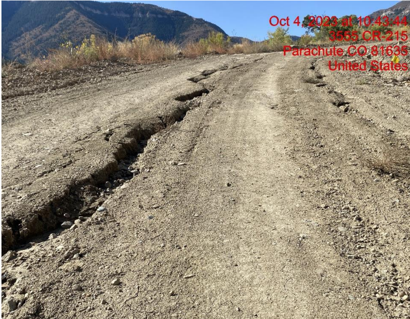
Insufficient Erosion Controls – Photo #06788
