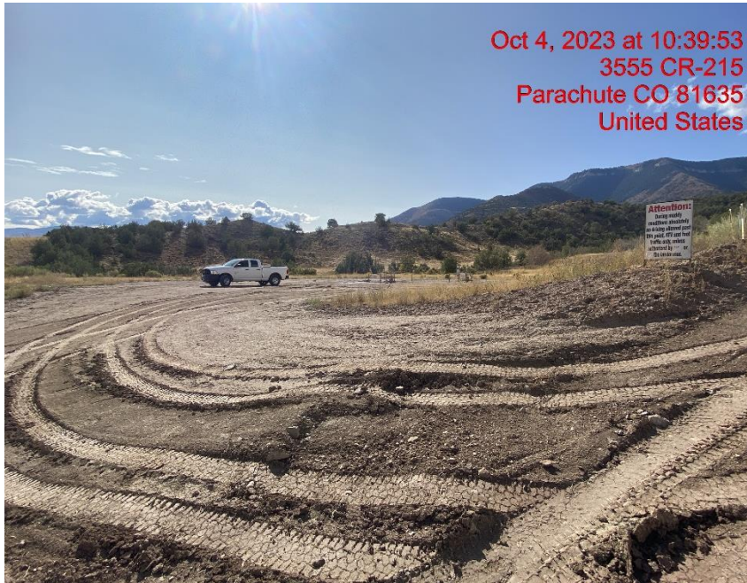
Lack of Stabilization/Insufficient Vehicle Tracking BMPs at Location Entrance/Exit – Photo #06784
