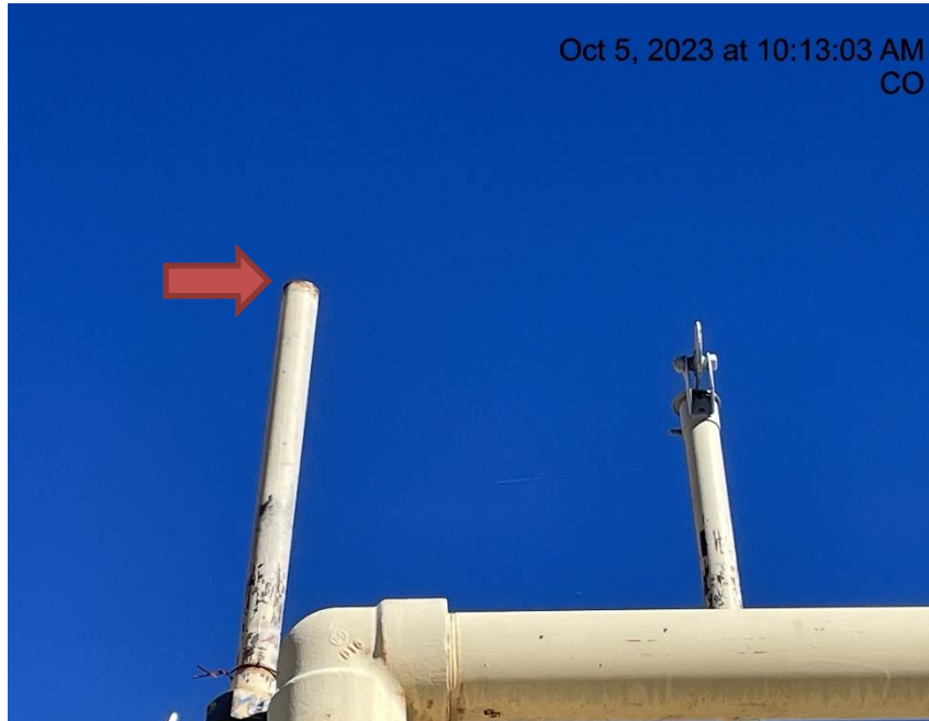
Photo # 1656 Rupture disc vent line lacks cap
