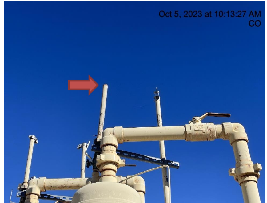
Photo # 1655 Rupture disc vent line lacks cap
