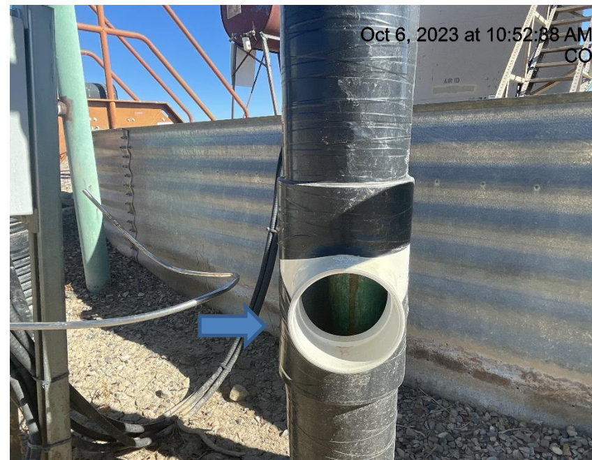
Photo # 1889 Flowline heating insulation open ended
