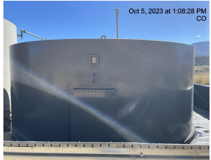
Photo # 1778 Production tank lacks required information
