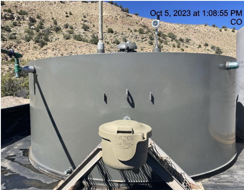
Photo # 1777 Production tank lacks required information
