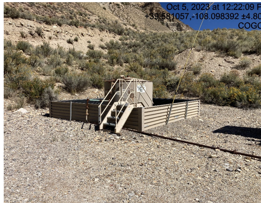
Tank battery lacking signage
