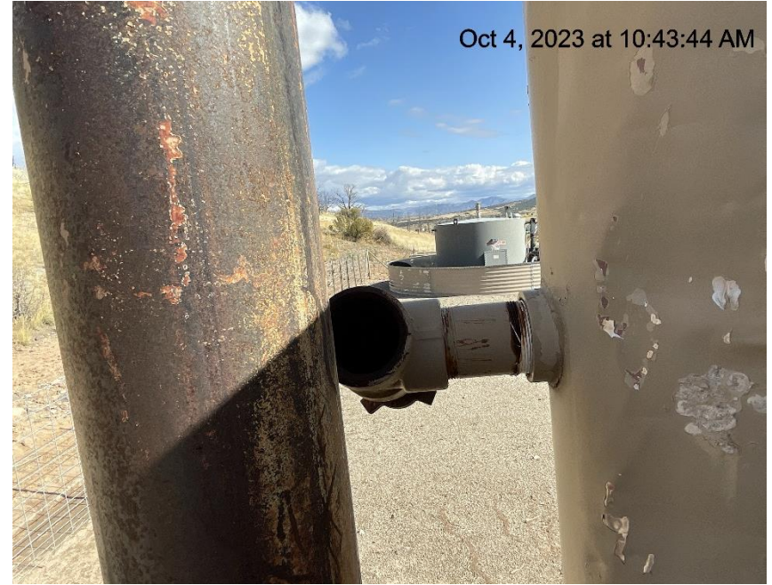
Photo # 1422 Open ended pipe/wildlife hazard
