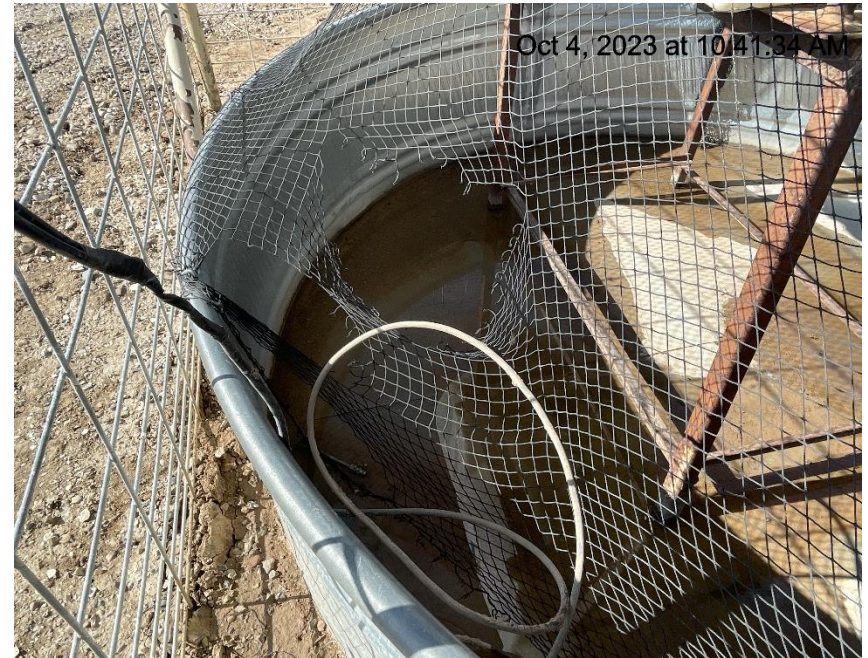
Photo # 1420 Netting/wildlife protection needs maintenance
