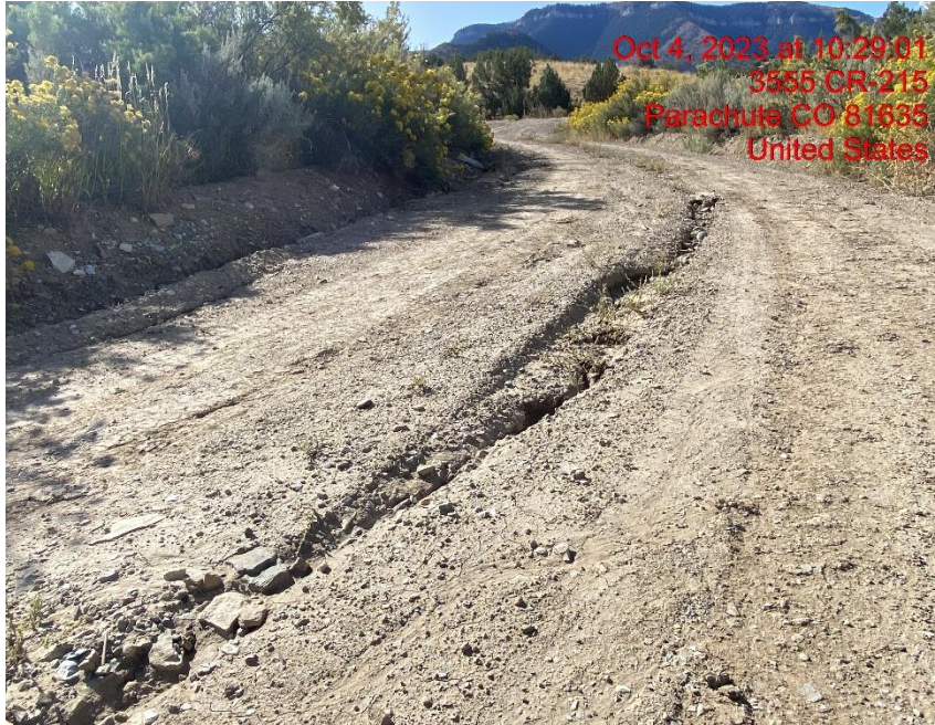
Rill Erosion Cutting Through Access Road – Photo #06774
