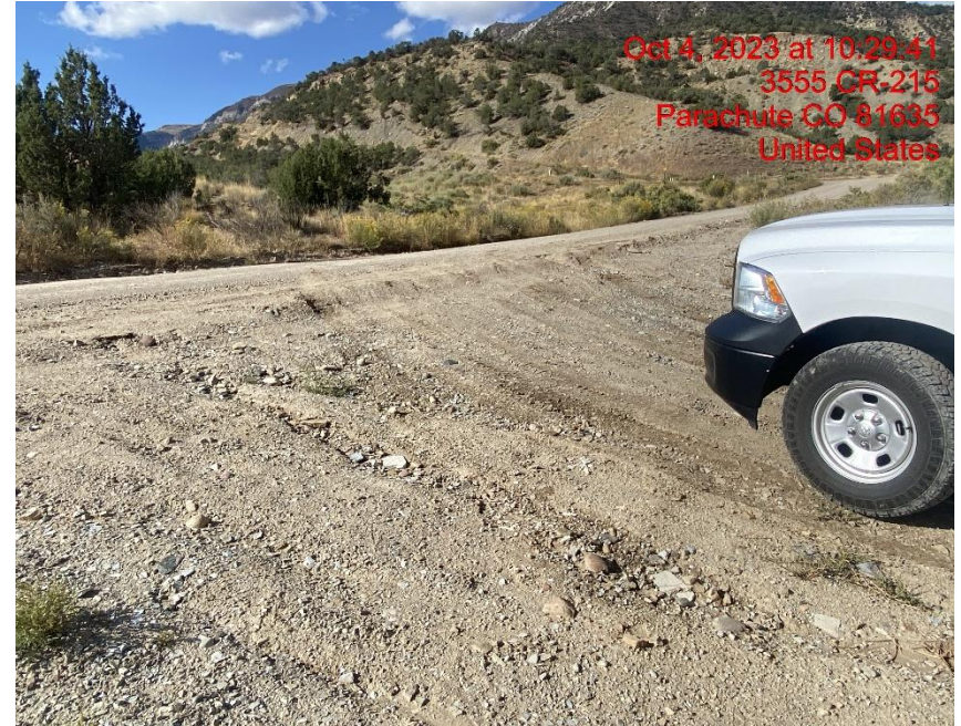
Insufficient Vehicle Tracking BMPs at Location Entrance/Exit – Photo #06775
