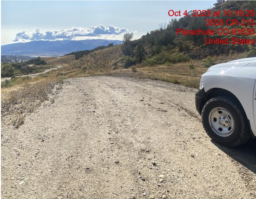
Insufficient Vehicle Tracking BMPs at Location Entrance/Exit – Photo #06763
