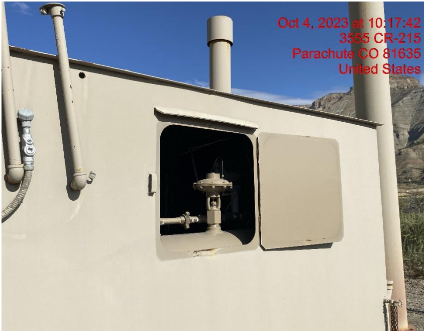
Unsecured Hatch on Separator – Photo #06759
