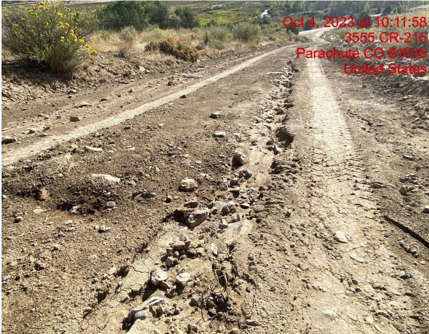
Rill Erosion Cutting Through Lease Road – Photo #06754
