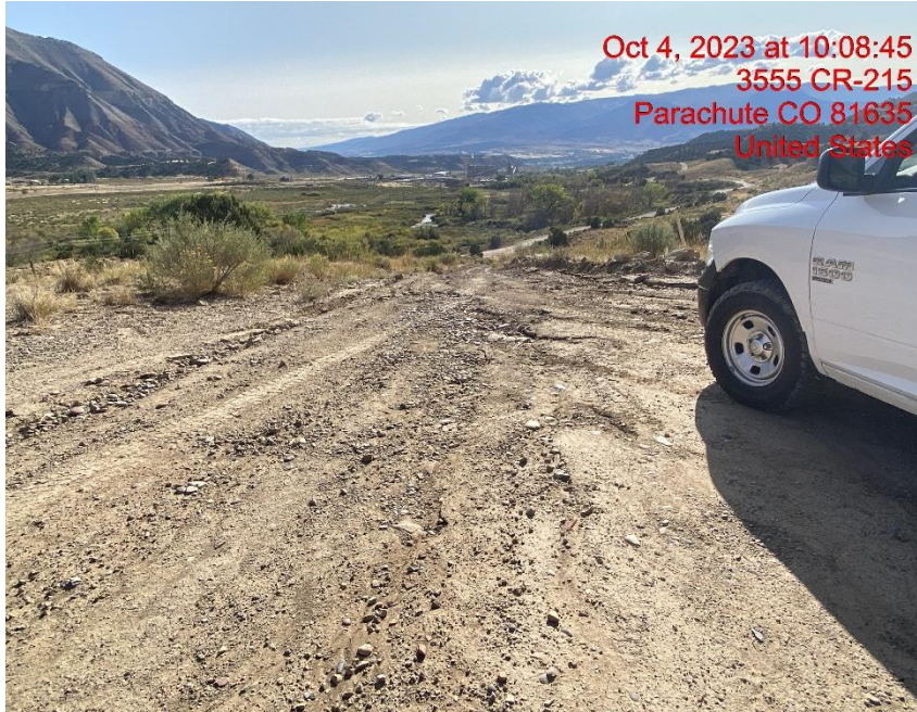
Insufficient Vehicle Tracking BMPs at Location Entrance/Exit – Photo #06752
