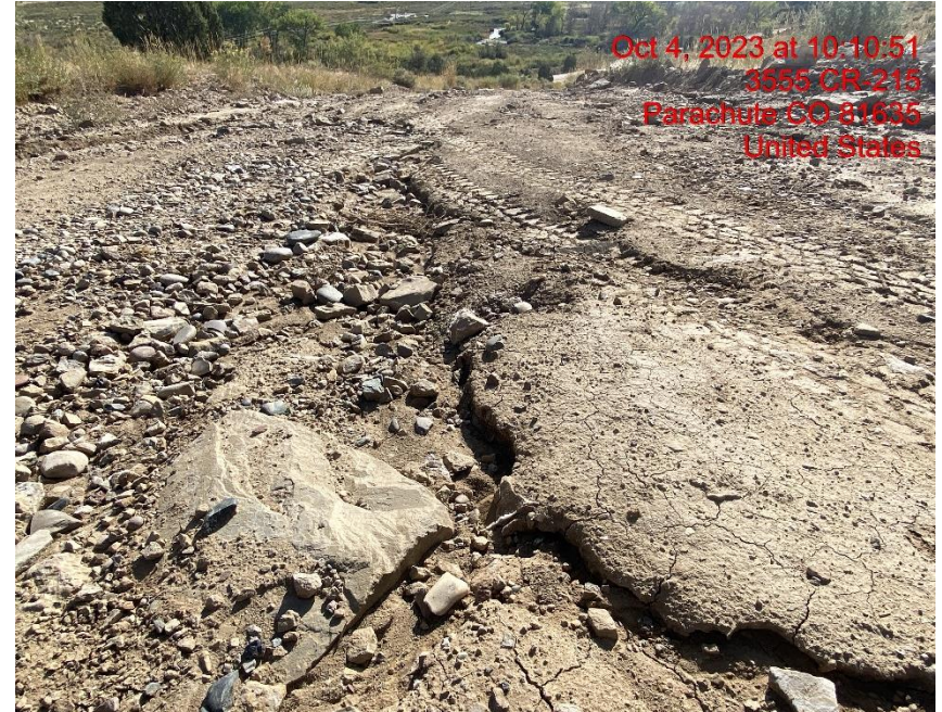
Rill Erosion Cutting Through Lease Road – Photo #06753
