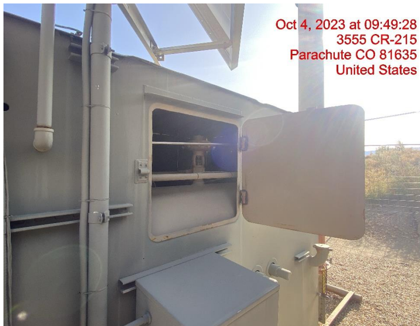
Unsecured Separator Hatch – Photo #06731
