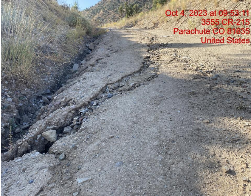
Rill Erosion Cutting Through Lease Road – Photo #06734
