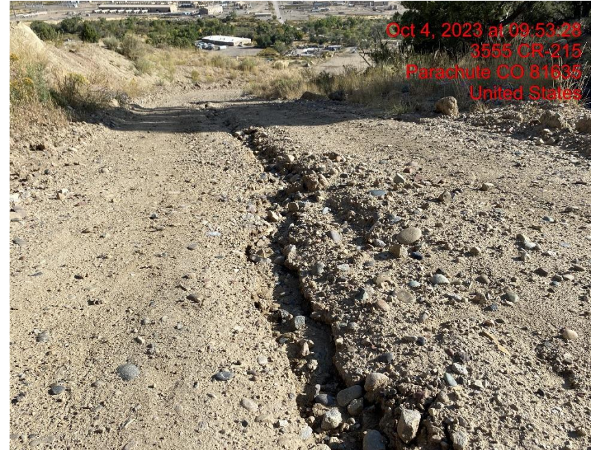
Rill Erosion Cutting Through Lease Road – Photo #06735
