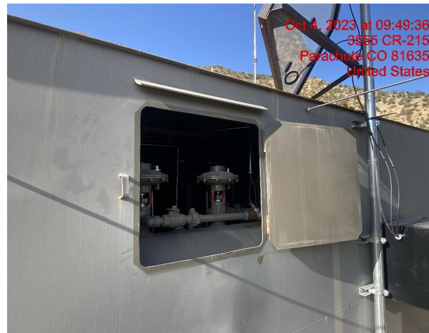
Unsecured Separator Hatch – Photo #06732
