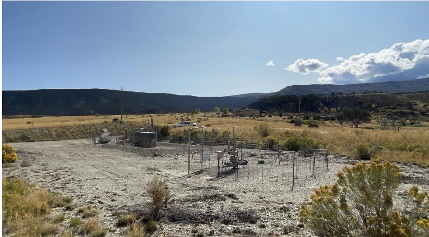
North West corner of location.
