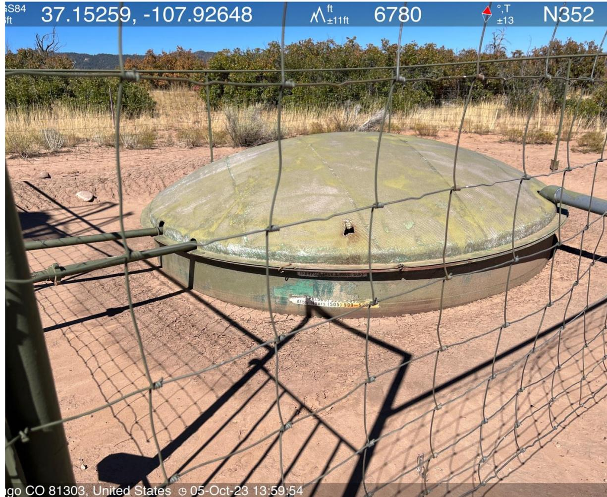
**Photo #6 View of non-legible labeling on the produced water tank.**
