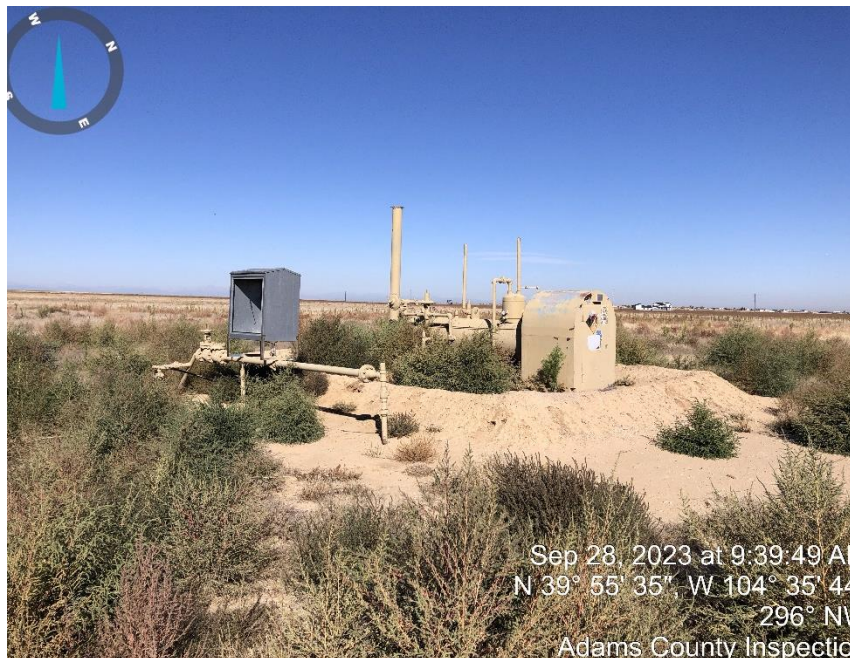
Photo #3 Separator, meter box & weeds throughout.
