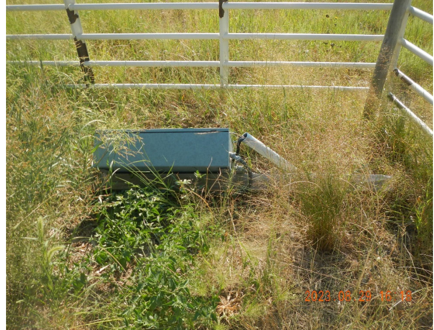
6. Downed Pump Jack Power and Control Panel. Note vegetation.
