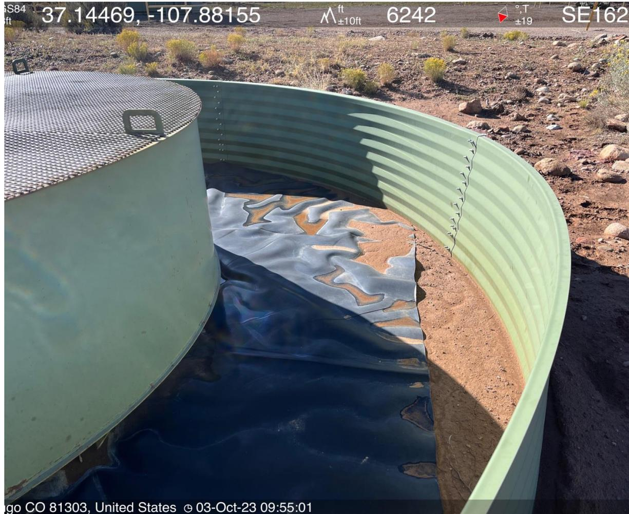
Photo #5 View of tank liner not covering entire base.
