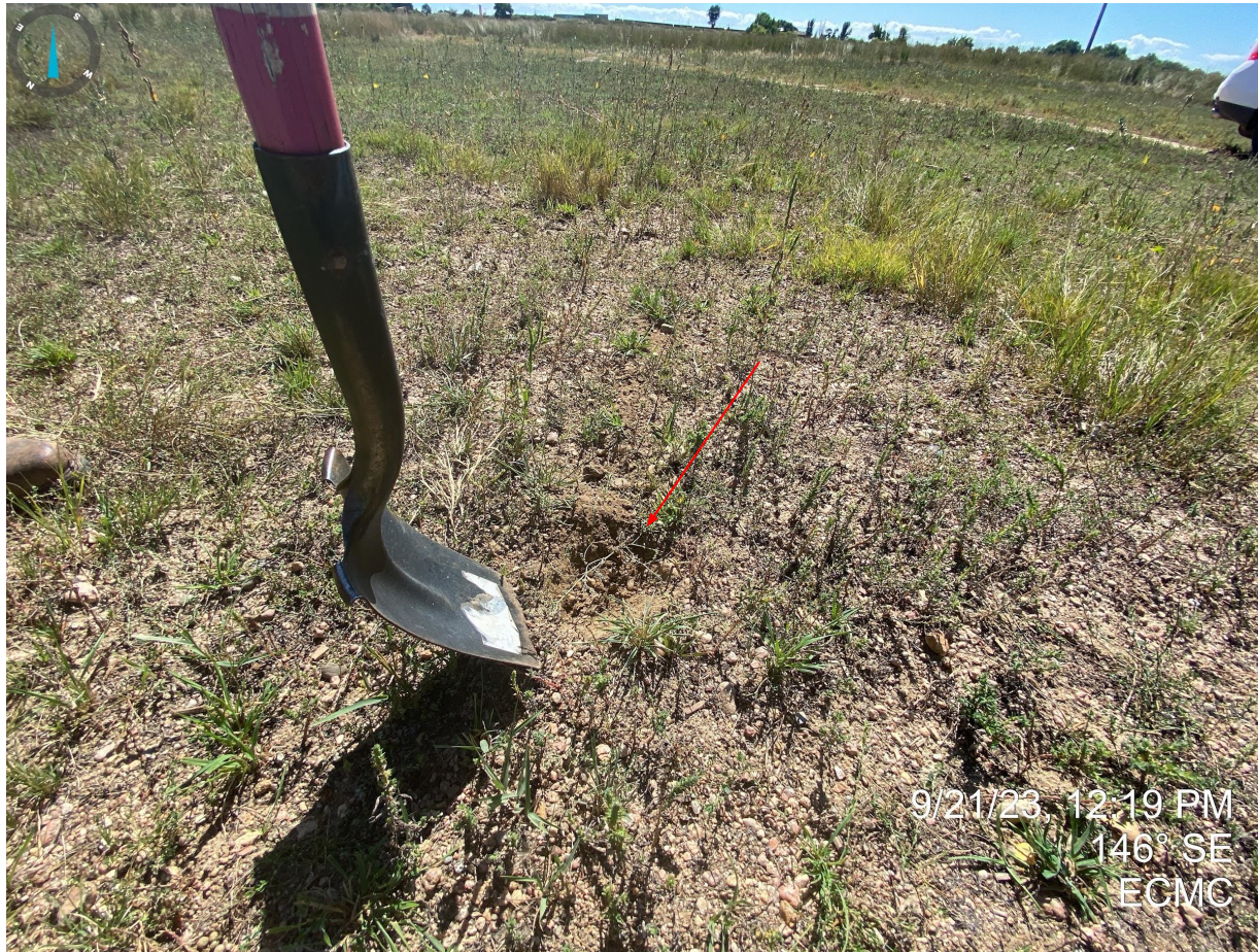
Photo 3. Taken within the former wellhead location. It does not appear the location was properly decompacted; hole is approximately 2-3" deep with road base/gravel present.
