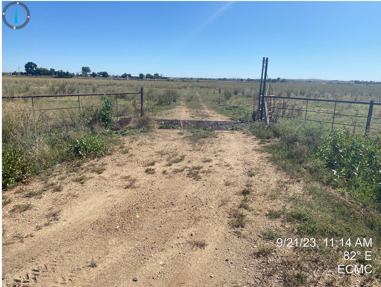
Photo 1. Taken near the entrance to the location. Photo illustrates that the approach/access road entrance has not been reclaimed and a cattle guard remains.
