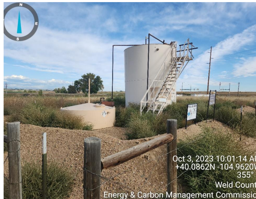
Photo 8 tank battery
