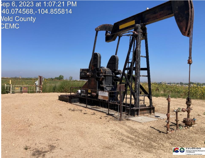
Pic 1 wellhead / pump jack
