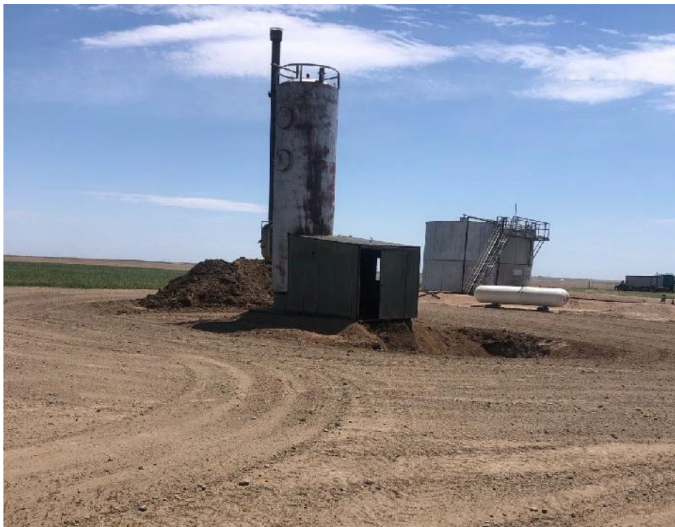
Photo after clean-up Wright Tank Battery (Looking Southeast)
