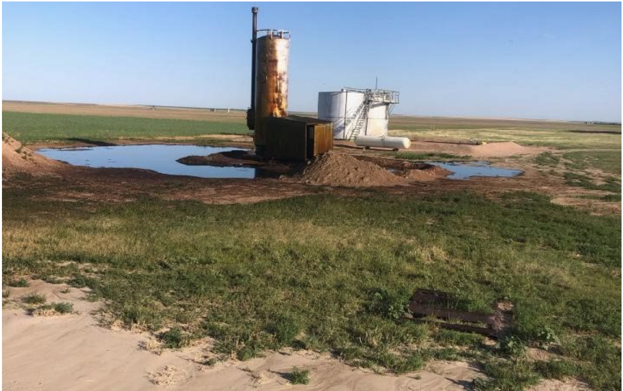
Initial spill photo Wright Tank Battery (WTB) July 2023 Spill
