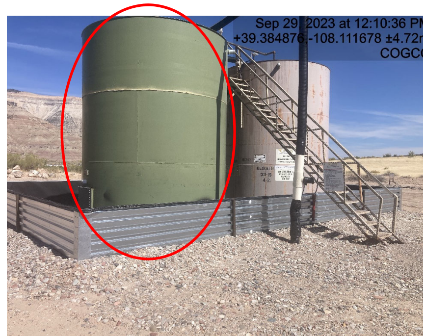
Tank is lacking labeling and lack of battery signage
