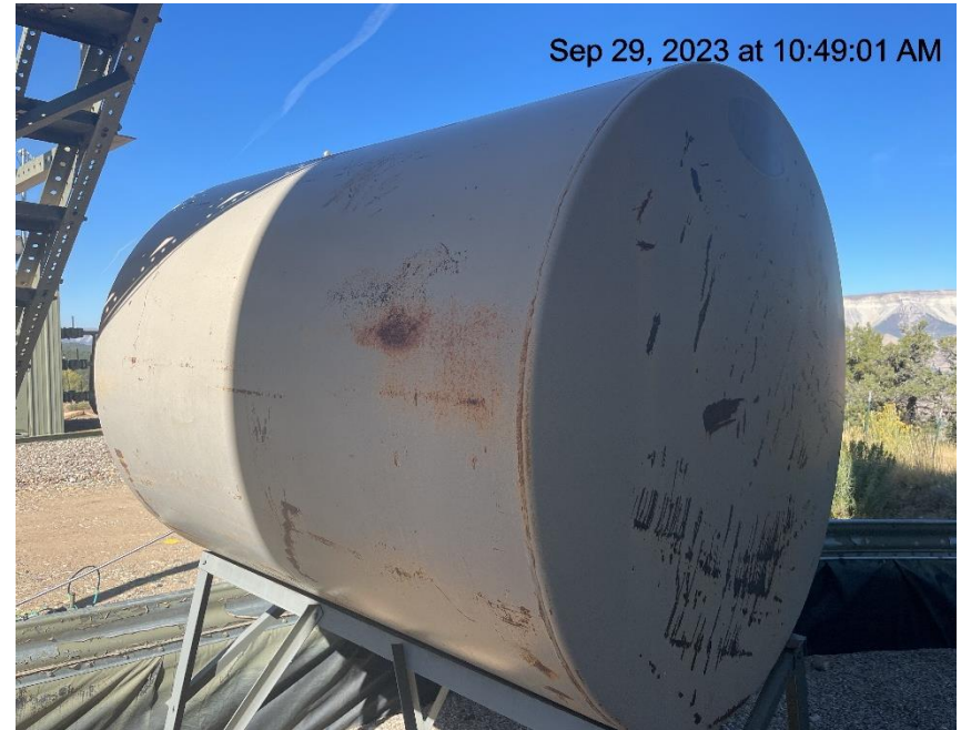
Photo # 1005 Methanol tank lacks required information
