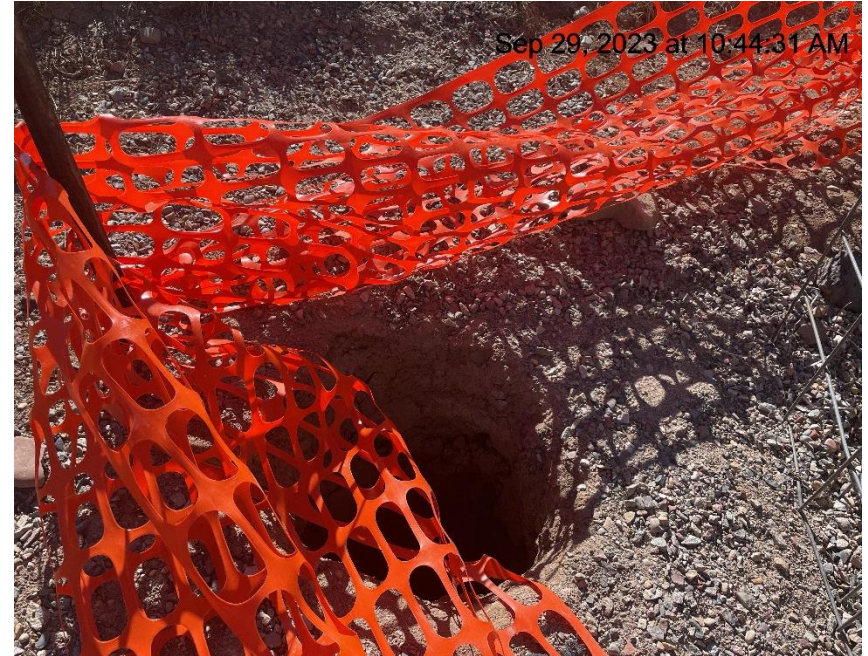
Photo # 1003 Construction barrier/wildlife protection needs maintenance
