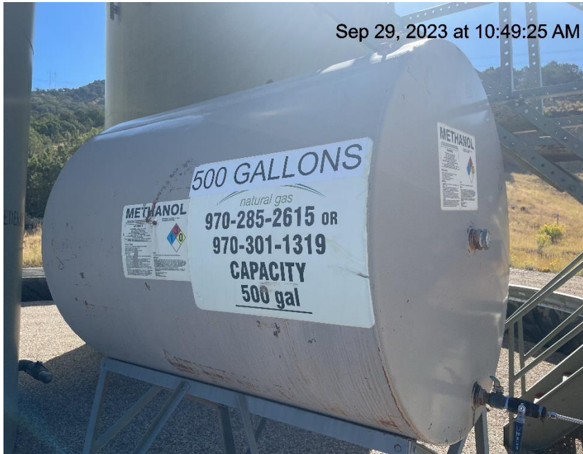
Photo # 1004 Methanol tank lacks required information
