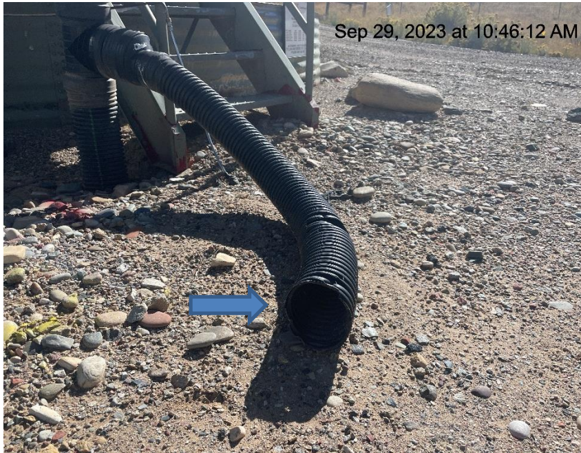
Photo # 1006 Flowline heating insulation open ended
