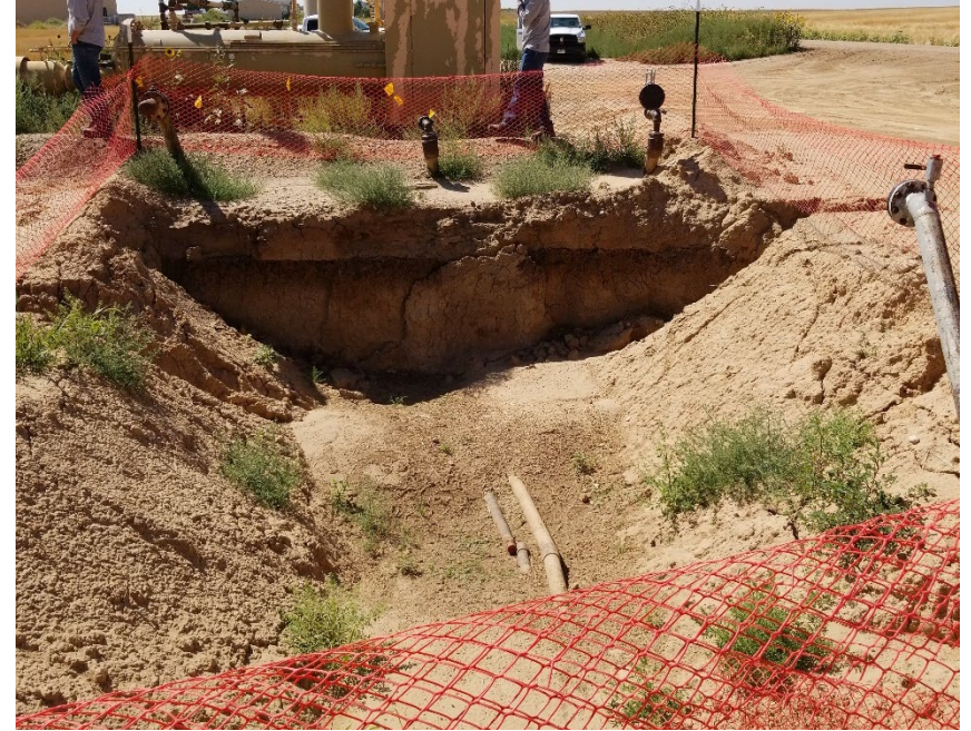
Excavation to expose the release point.
