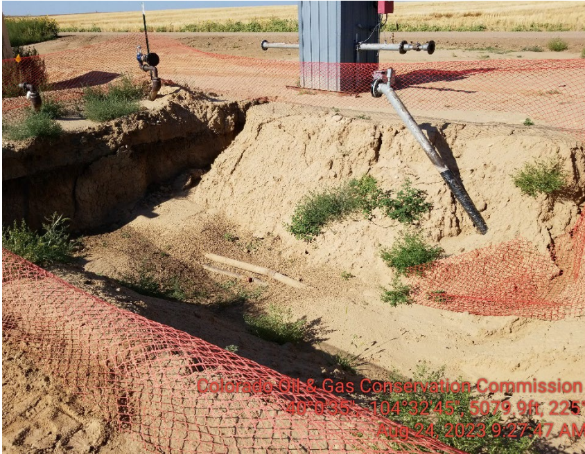
Excavation to expose the release point.
