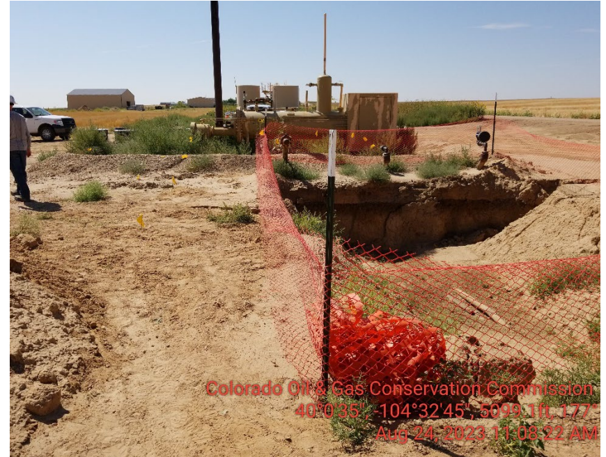
Excavation to expose the release point.
