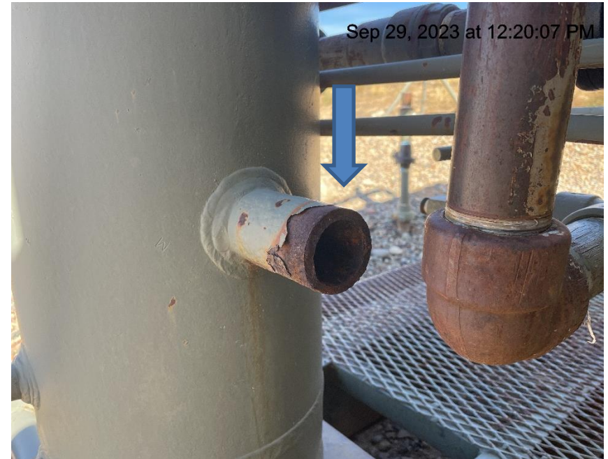
Photo # 1153 Open ended pipe on production unit
