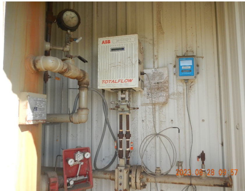
6. Vertical separator and digital gas meter run.
