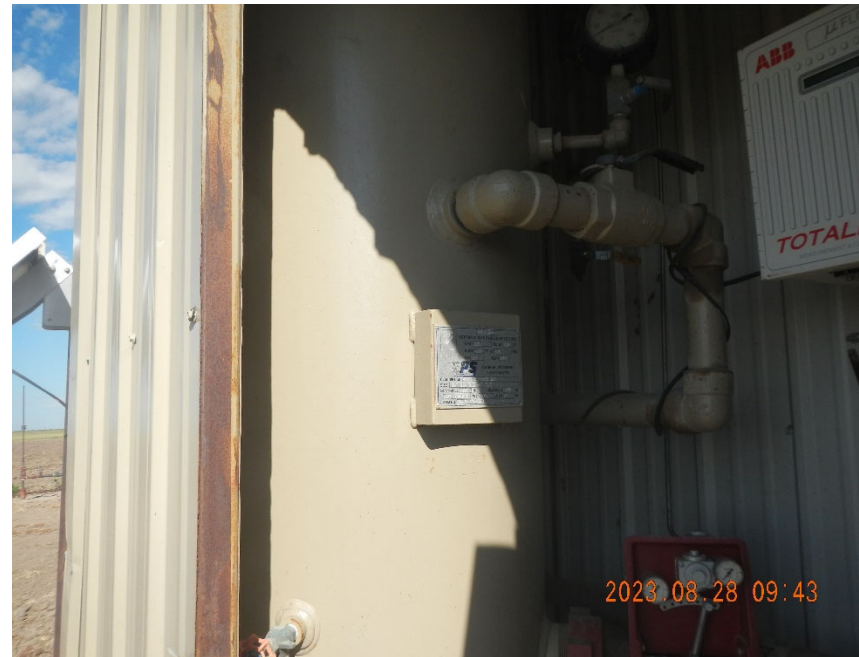
6. Vertical separator inside meter shed.
