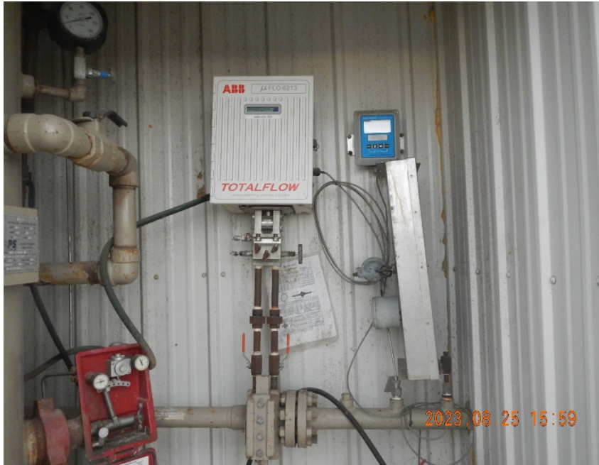
7. Digital gas meter run.
