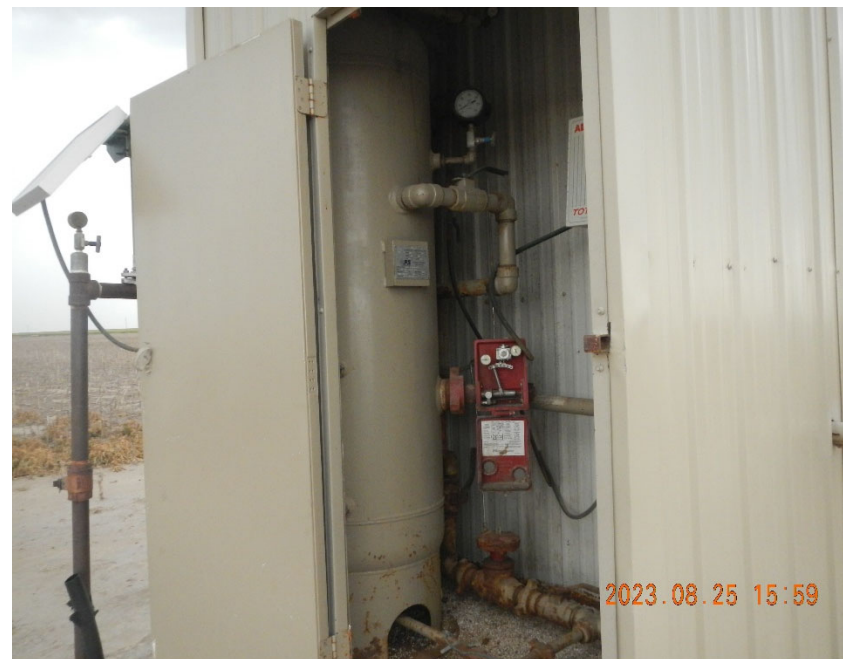
6. Vertical separator inside meter shed.
