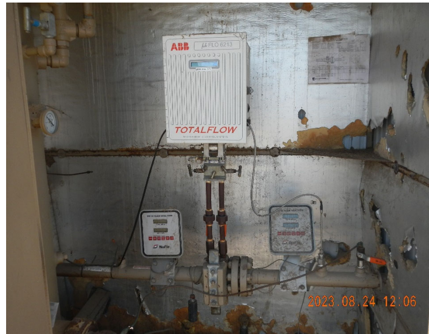
8. View of digital gas meter run.
