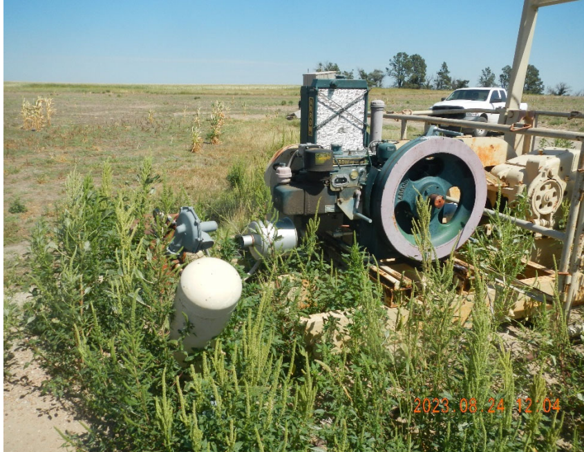
5. Prime mover and supply gas vessel. Noted vegetation.
