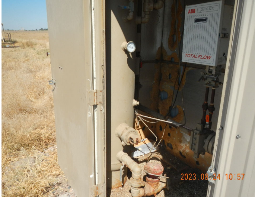
9. Vertical separator inside meter shed.
