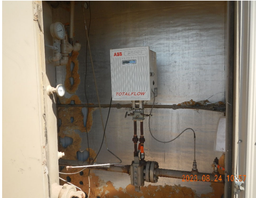
7. View of digital gas meter run.
