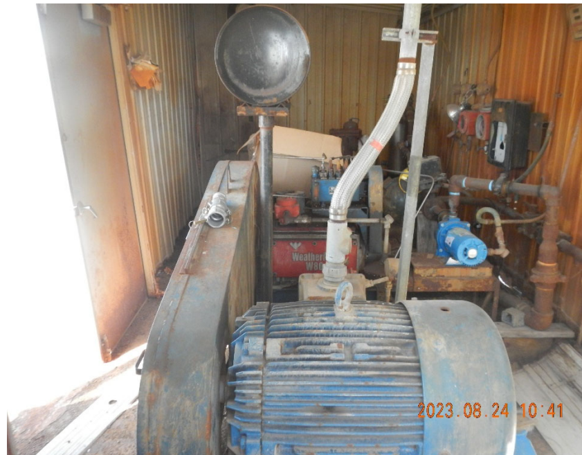
4. Electric injection pump.
