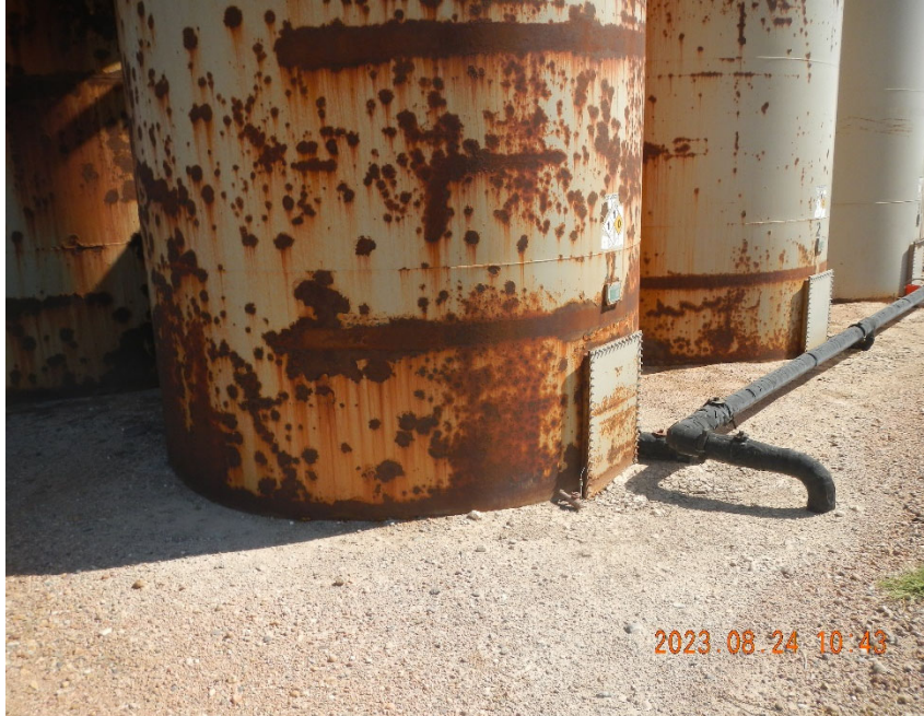
9. Tank with rust, pitting, and peeling paint in need of inspection and repair.
