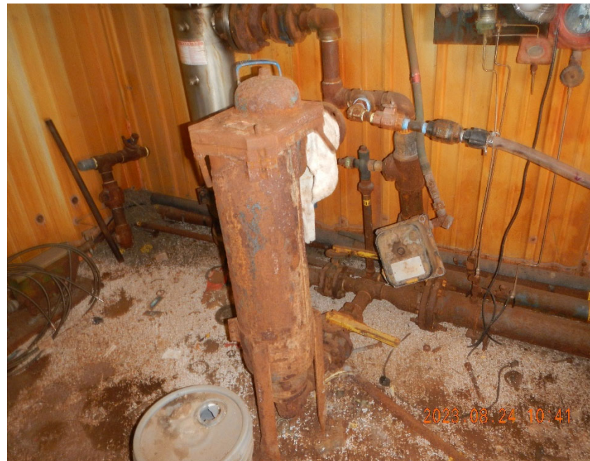
6. Produced water filter.
