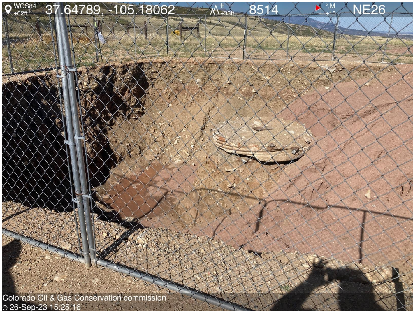
PHOTO 3: It appears the well was plugged and abandoned on 8/9/2022. There is an open excavation at the wellhead from an active remediation that is still ongoing. The wellhead will need to be cut and capped deep enough to allow recontouring back to the original grade. Comply with 1004 Rules
