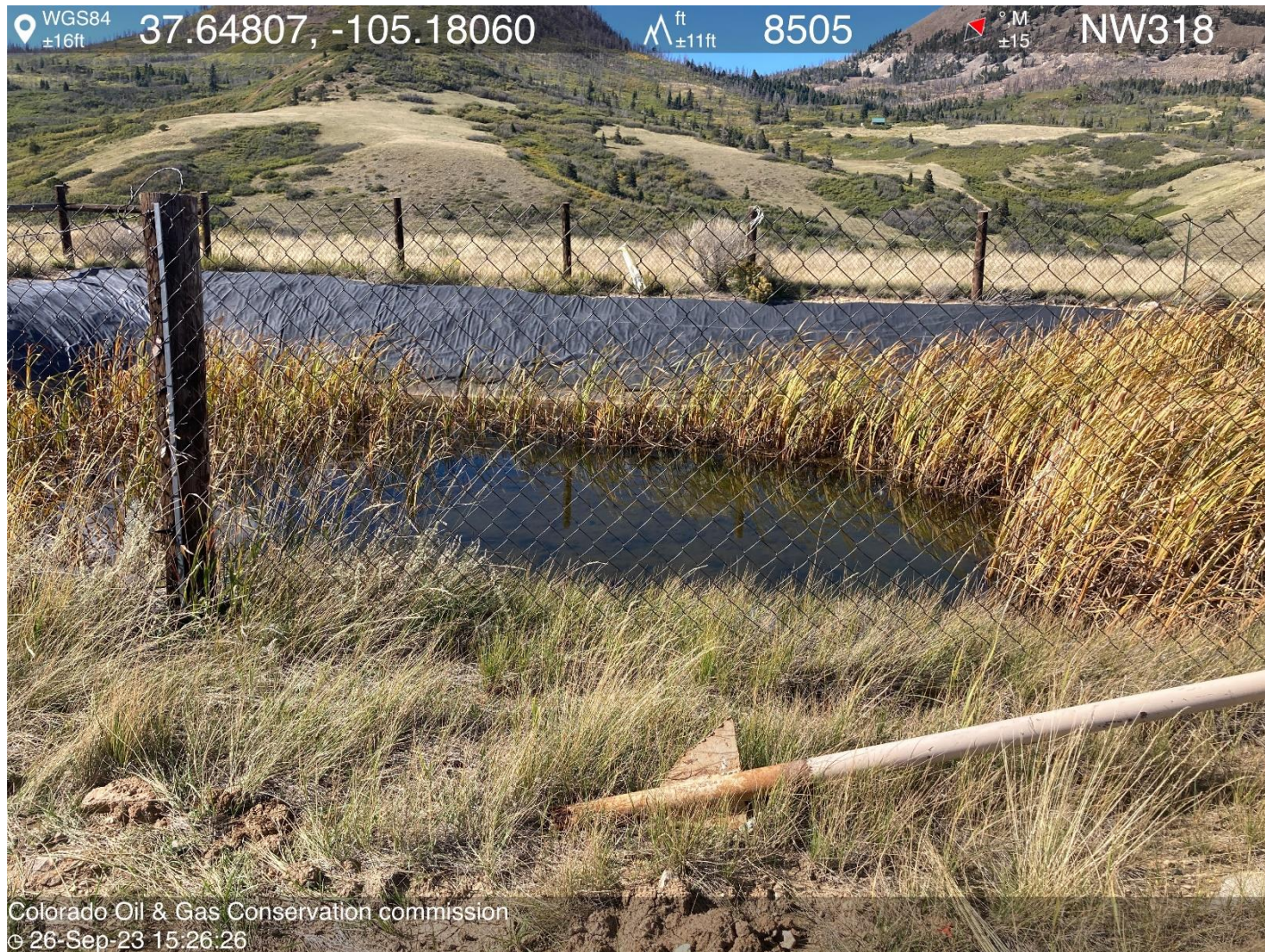
PHOTO 3: There is a lined pit at the wellsite that should have been closed within 3 months of abandonment (11/9/2022). Comply with 1004 Rules
