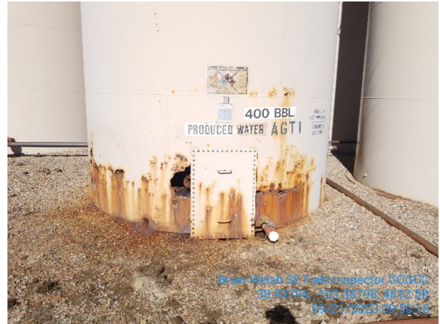
AGT 1 water tank is rotted out and needs removed
