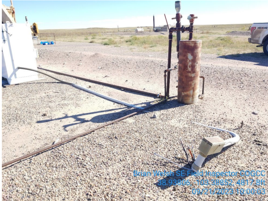
Electrical wires exposed
