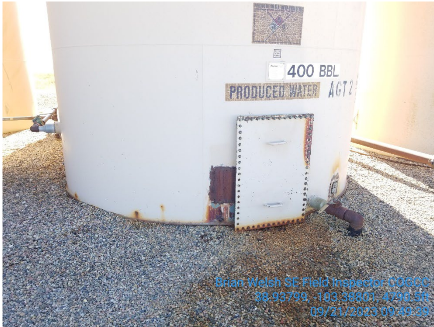
AGT 2 water tank has leaking rust spots
