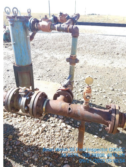
This water transfer pipe has a hole and needs repaired
