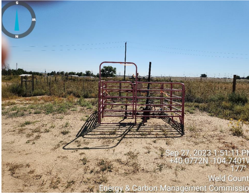
Photo 1 well head and equipment
