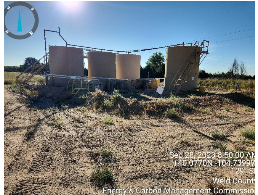
Photo 14 tank battery
