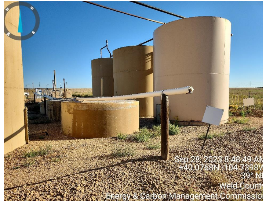
Photo 12 tank battery
