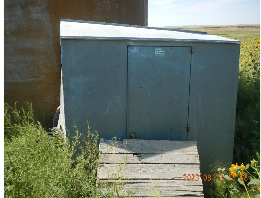
6. Equipment Shed inside bermed area.
