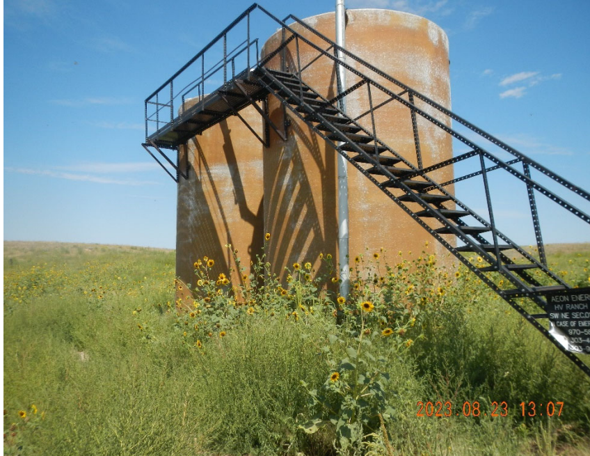
3. View of tank area. Note vegetation.
