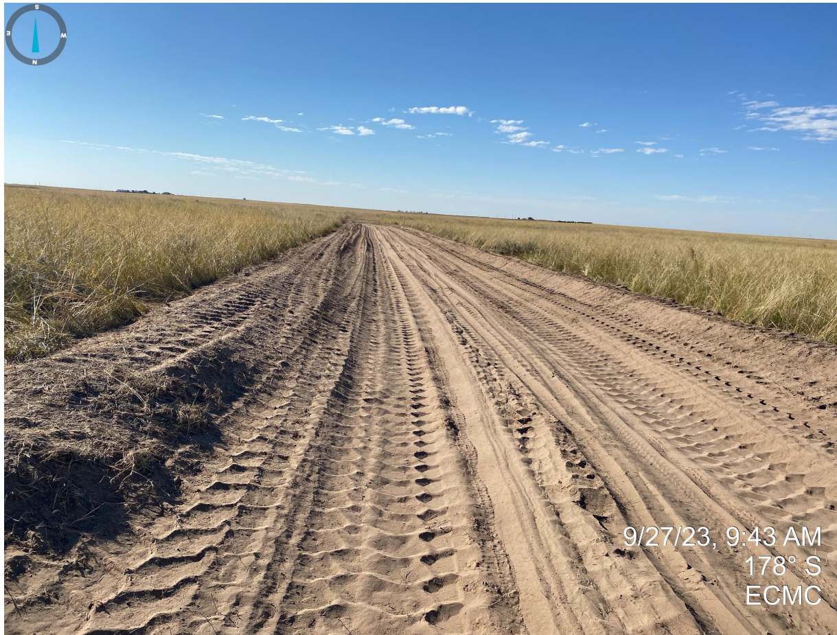
Photo 2. Taken south of the location entrance. It appears the access road has had topsoil salvaged and stored on the sides of the road. Additional BMPs are required to stabilize the stockpiled soils as wheel packing alone is not adequate due to the site conditions.
