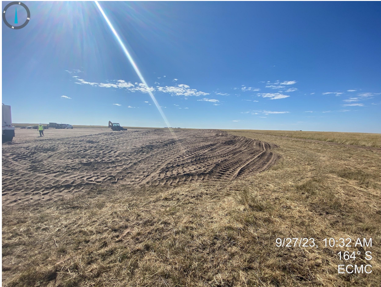
Photo 10. Taken near the northwest corner of the location, facing the topsoil stockpile. Additional BMPs are required to stabilize the stockpiled soils as wheel packing alone is not adequate due to the site conditions.
