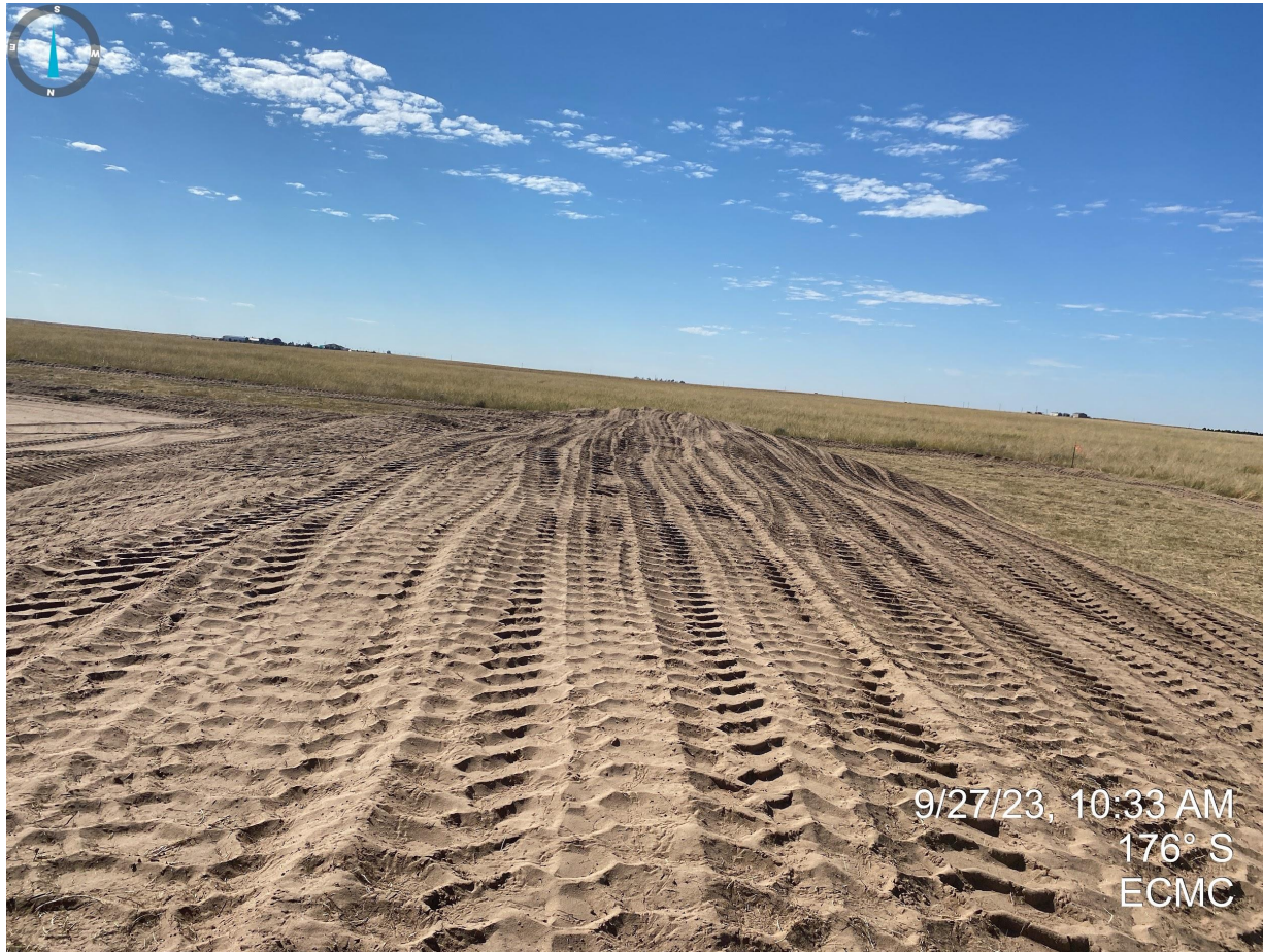
Photo 12. Taken from the middle portion of the topsoil stockpile. Additional BMPs are required to stabilize the stockpiled soils as wheel packing alone is not adequate due to the site conditions.
