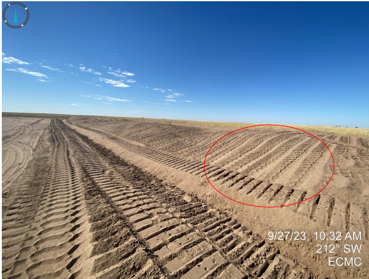
Photo 11. Taken from the northern portion of the topsoil stockpile. Wheel packing marks are parallel to the slope as opposed to perpendicular. Additional BMPs are required to stabilize the stockpiled soils as wheel packing alone is not adequate due to the site conditions.
