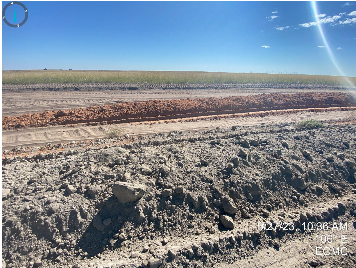
Photo 14. Taken from the eastern portion of the pad. Appears material is being brought in to stabilize the drilling pad.
