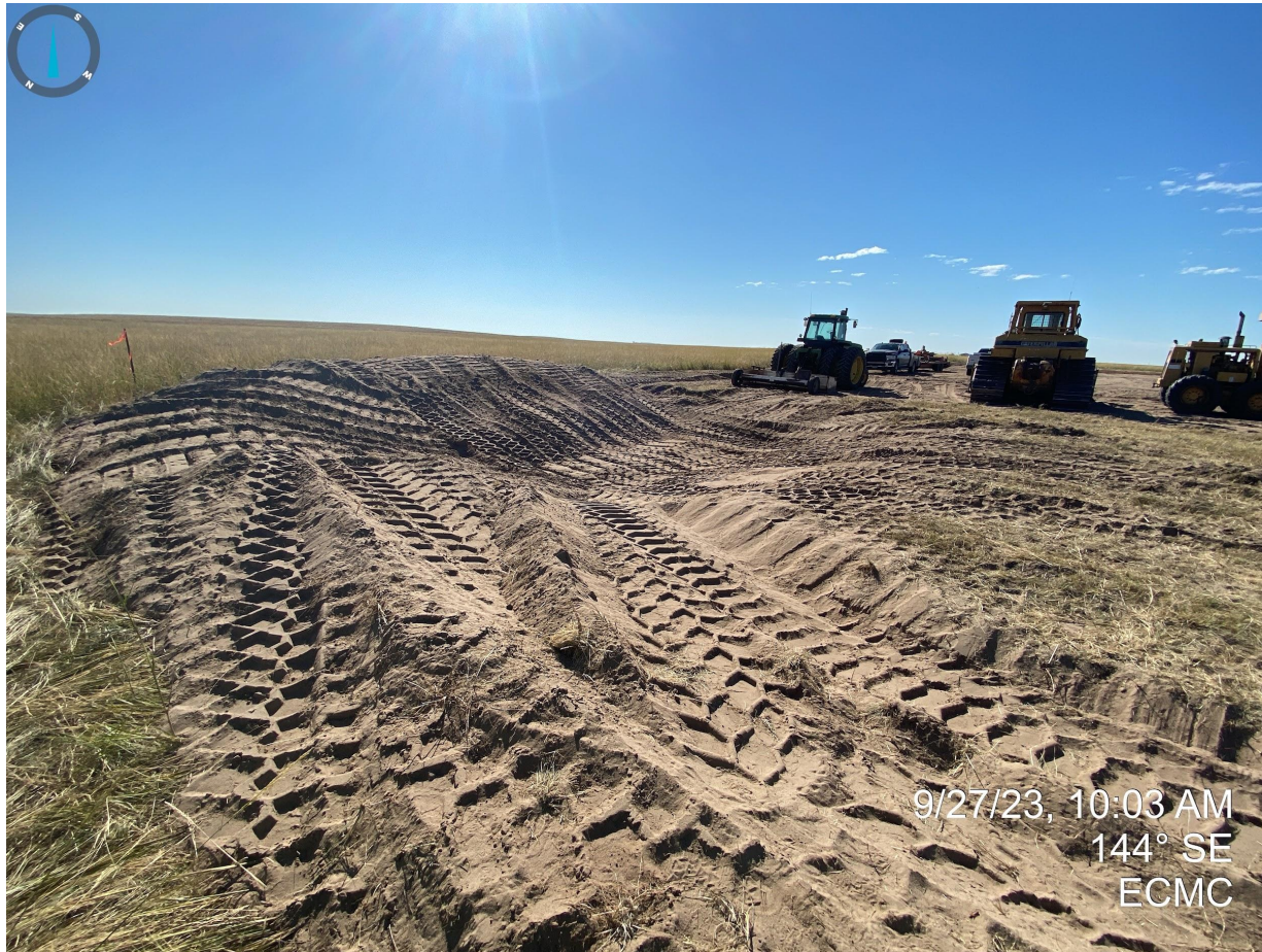
Photo 4. A sediment trap was installed on the northeast corner of the location. The sediment trap and berm material are comprised of unstabilized material and require additional BMPs to protect against wind and water erosion degradation, as wheel packing alone is not adequate due to the site conditions.
