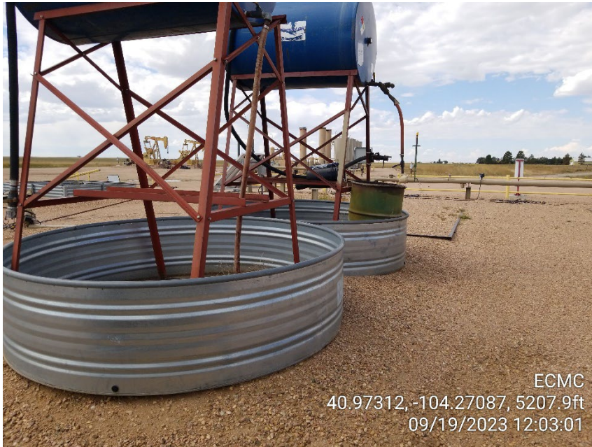
Photo 3 – Wildlife Netting missing from Day Tank Secondary Containments
