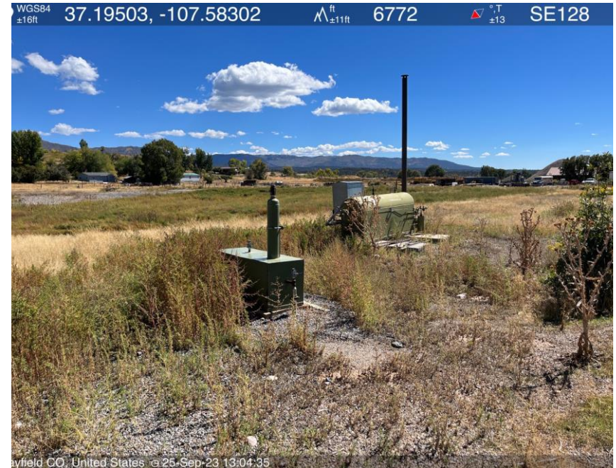
Photo #6. View of corrective action not completed. Weeds growing around wellhead, separator, and across location.
