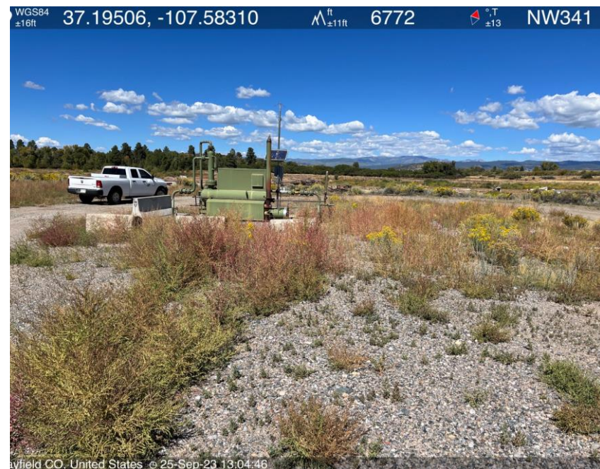
Photo #2. View of corrective action not completed. Weeds growing around separator, wellhead, and across location.
