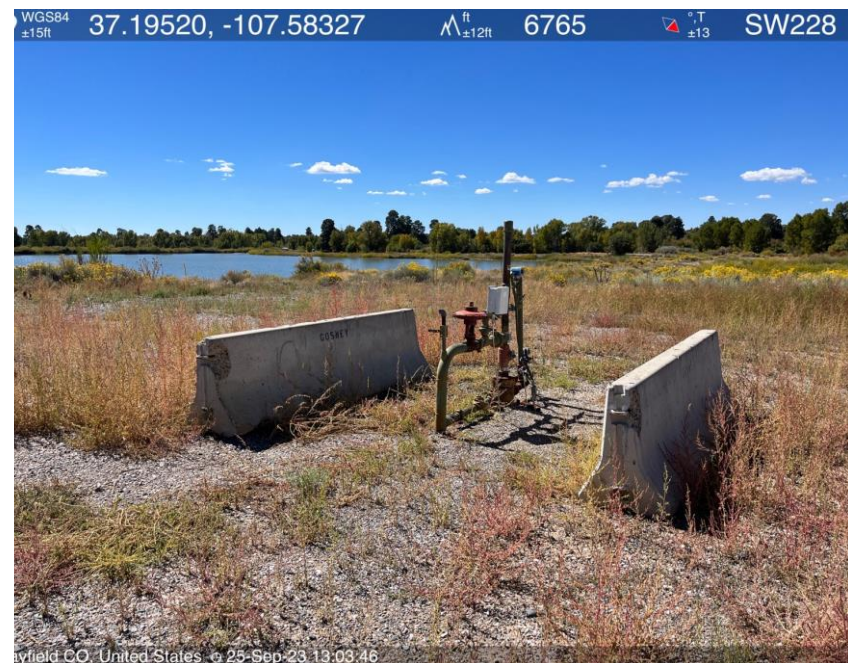
Photo #4. View of corrective action not completed. Weeds growing around wellhead, separator, and across location.
