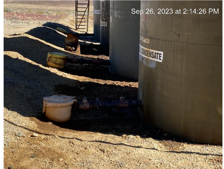
Staining all around tank battery
