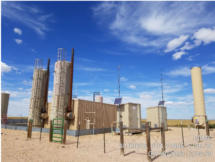
Photo 1 – Heater Treaters, Gas Meters and ECD
