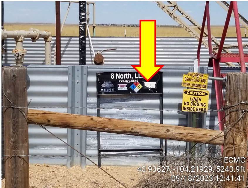
Photo 3 – Capacity Label missing
