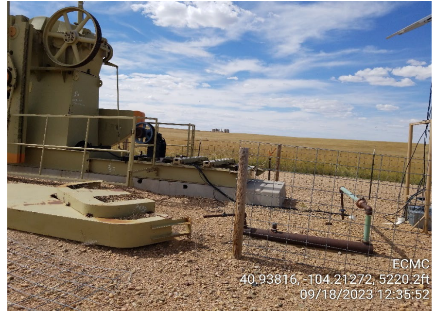
Photo 4 – Engine and Housing Removed
