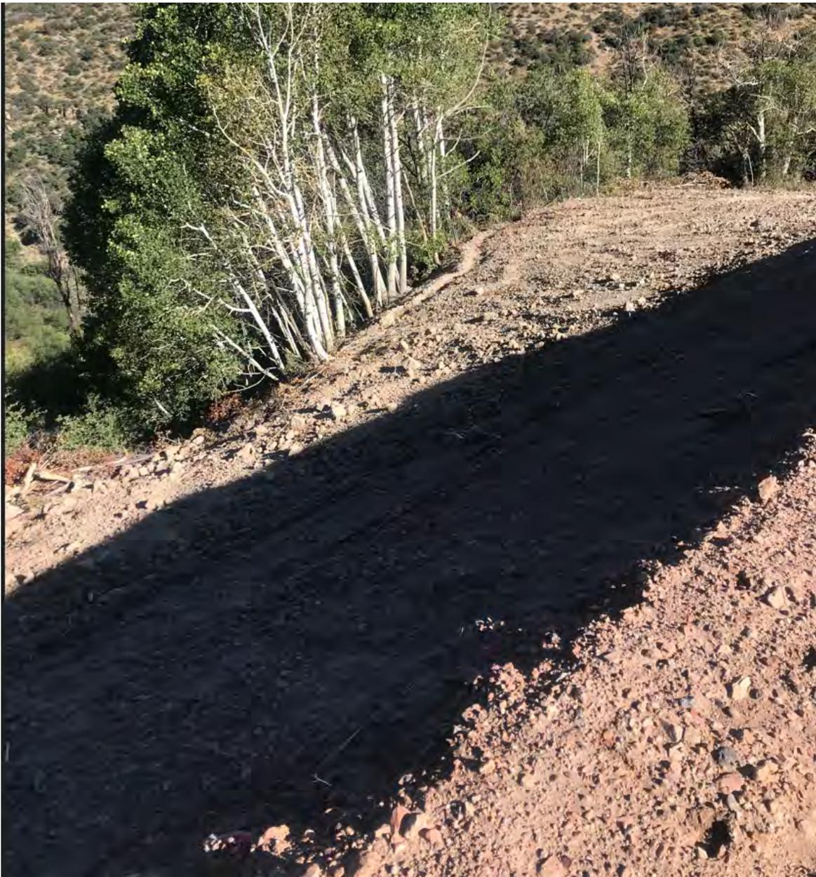
Wattles have been installed and spoil piles that were present downslope of the wattle have been removed.
