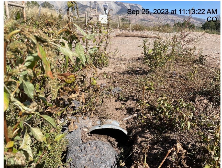
Photo # 623 Culvert needs maintenance (near wellhead)
