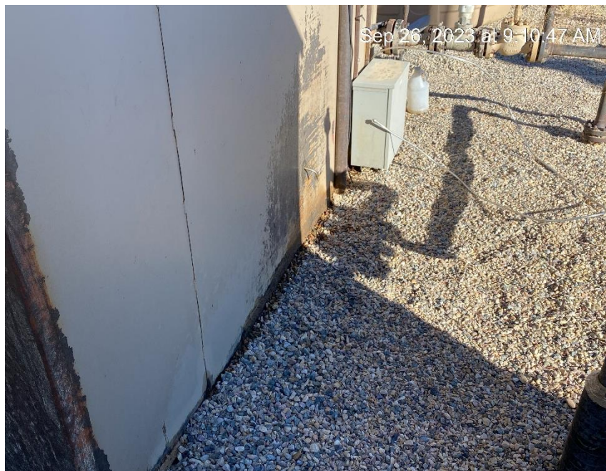
Staining from inside leaks
