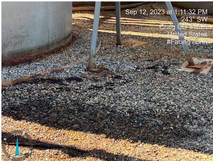
Photo 53 and 54. Photo taken of stained soils within secondary tank containment on southeast Location (left); stained soils on working pad area (right).
