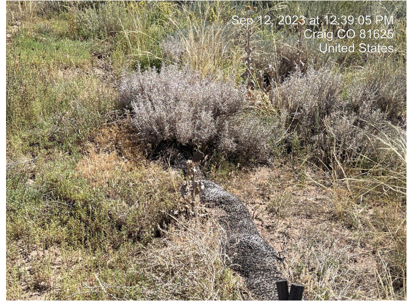
Photo 13 and 14. Wattles at the south end of the fill slope, which have deteriorated and are considered debris.
