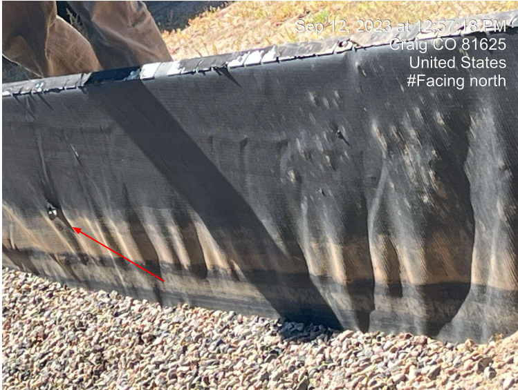
Photo 45 and 46. Photo taken of secondary containment on eastern edge of Location. Liner and metal containment contains a puncture mark.
