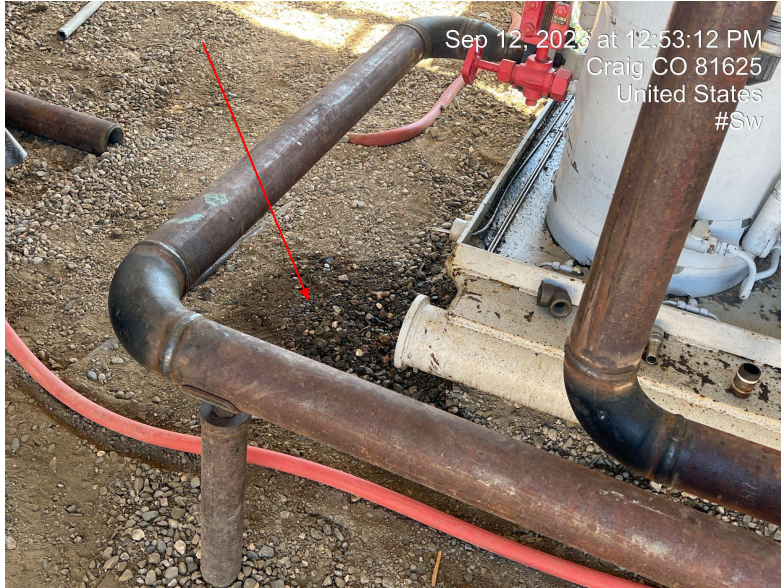
Photo 39 and 40. Stained soils found within shed underneath pipe (left) and underneath engine oil tank (right).
