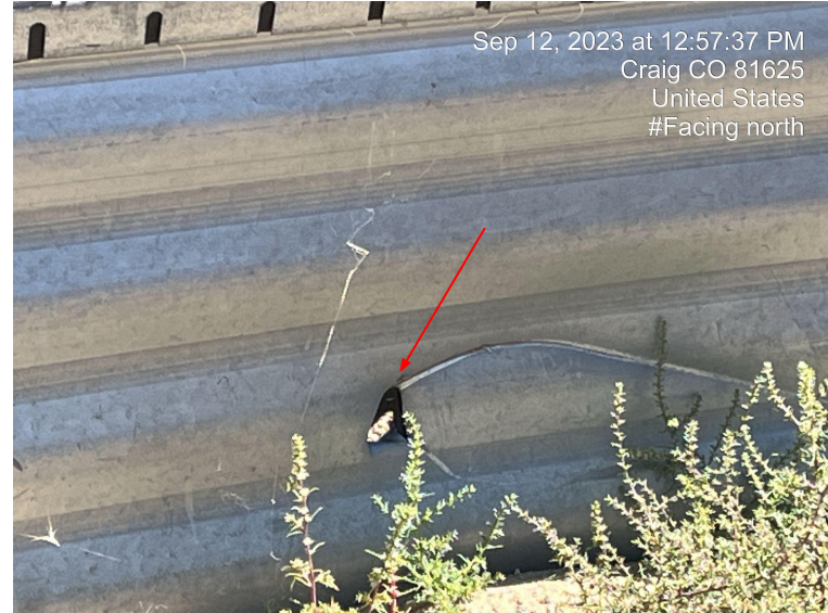
Photo 45 and 46. Photo taken of secondary containment on eastern edge of Location. Liner and metal containment contains a puncture mark.
