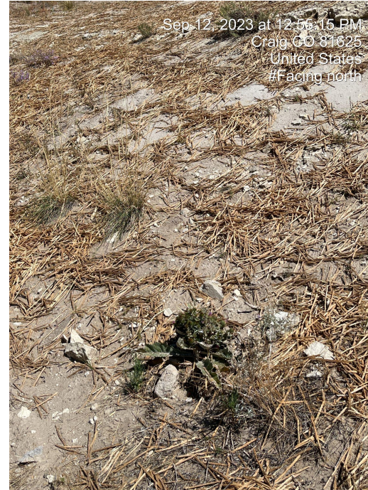
Photo 43 and 44. Photo taken of cut slope on eastern edge of Location; wood straw used for stabilization.
