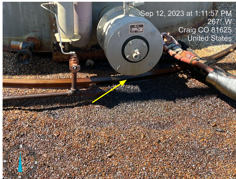
Photo 51 and 52. Photo taken of stained soils within secondary tank containment on southeast Location; active leak from tank (right).
