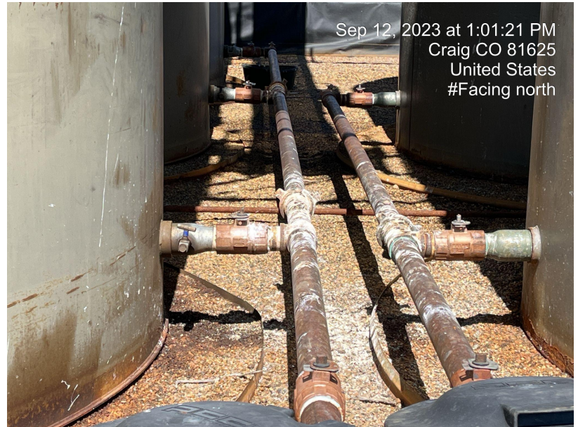
Photo 47 and 48. Photo taken of stained soils within secondary tank containment on southeast Location.
