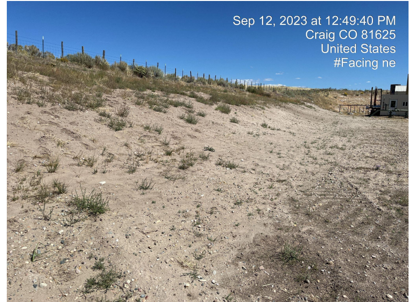
Photo 29 and 30. Overview of cut slope on western edge of Location. It appears that the slope was temporarily tracked, but has no additional soil stabilizing BMPs.
