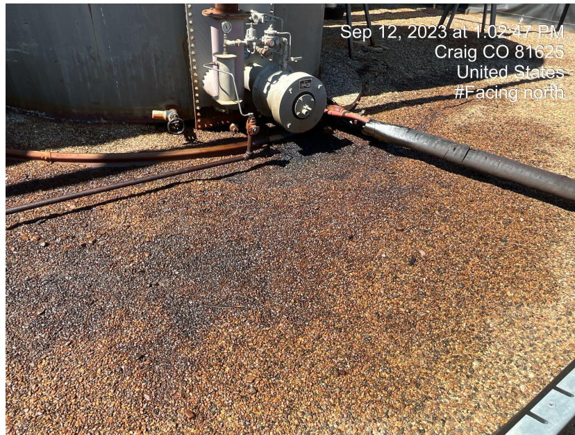
Photo 49 and 50. Photo taken of stained soils within secondary tank containment on southeast Location; active leak from tank (right).
