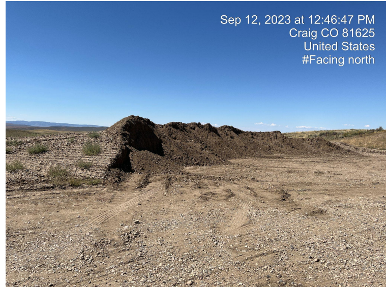
Photo 23 and 24. Photo taken of the stockpiled soil on the western edge of the working pad area. Operators were in process of removing soil for use on pad.
