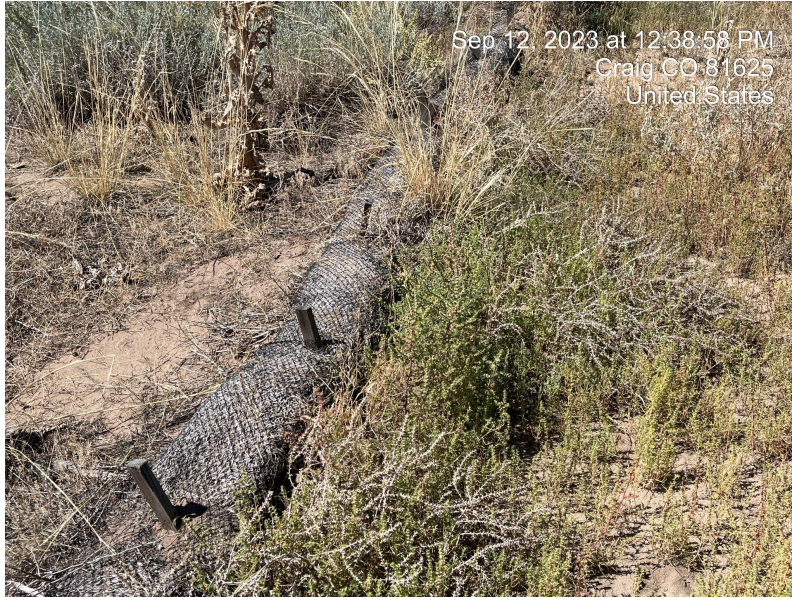
Photo 13 and 14. Wattles at the south end of the fill slope, which have deteriorated and are considered debris.
