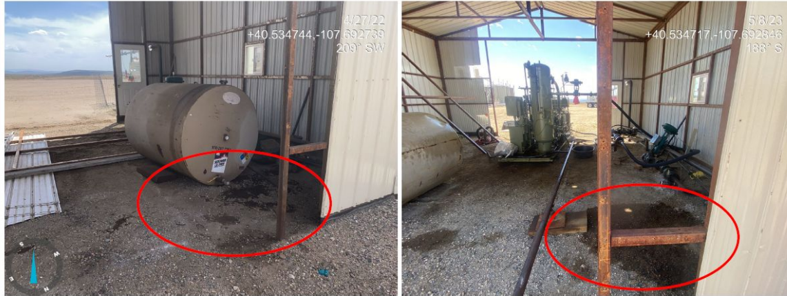
Photo 10. Photos show stained soils and unused equipment and debris throughout the shed Located at the northeast of the Location. Note the staining within the shed (circled) has increased in size and coverage since from the 4/27/22 inspection (left) to the current 5/8/23 inspection (right).
