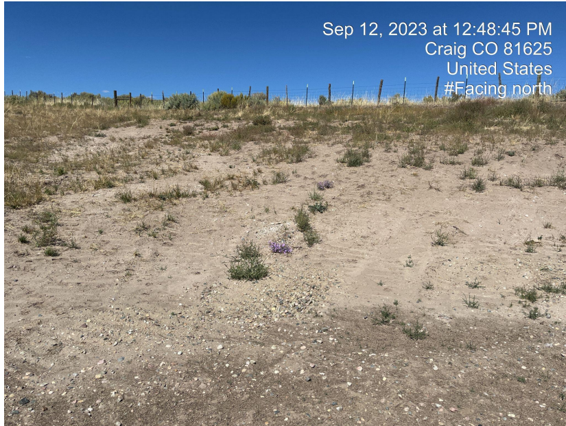
Photo 29 and 30. Overview of cut slope on western edge of Location. It appears that the slope was temporarily tracked, but has no additional soil stabilizing BMPs.
