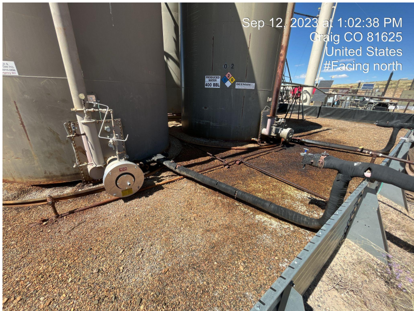
Photo 49 and 50. Photo taken of stained soils within secondary tank containment on southeast Location; active leak from tank (right).
